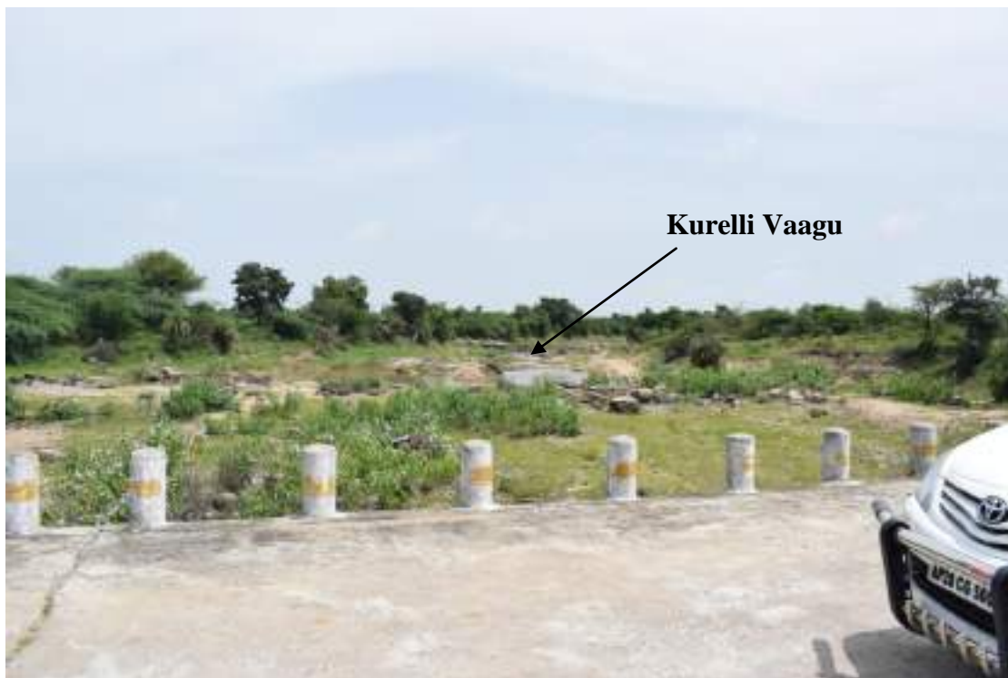
Photo 3: Existing bridge on Kurelli Vaagu stream.
