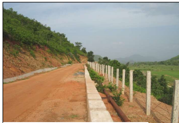
Inspection road and garland drain
