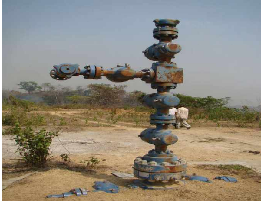
Fig. 4. GOAB-gas bearing well
