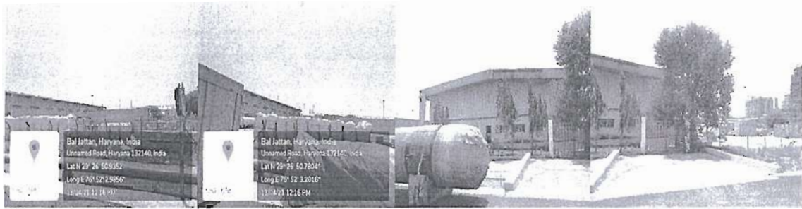
Photo 4: Part of proposed expansion site of Polypropylene plant
