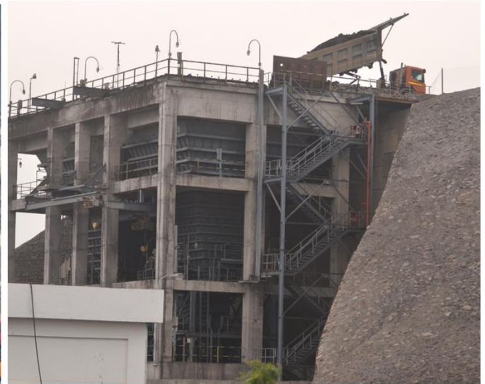
Unloading of trucks
