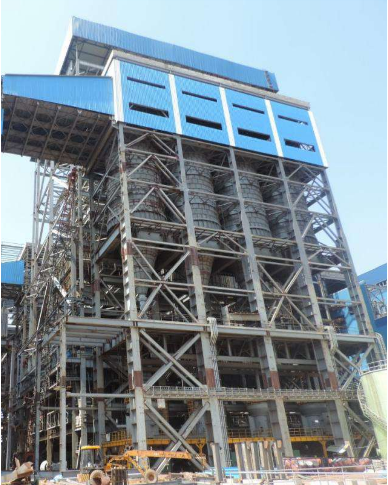
Bunker # 1A – Painting and cladding work in progress
