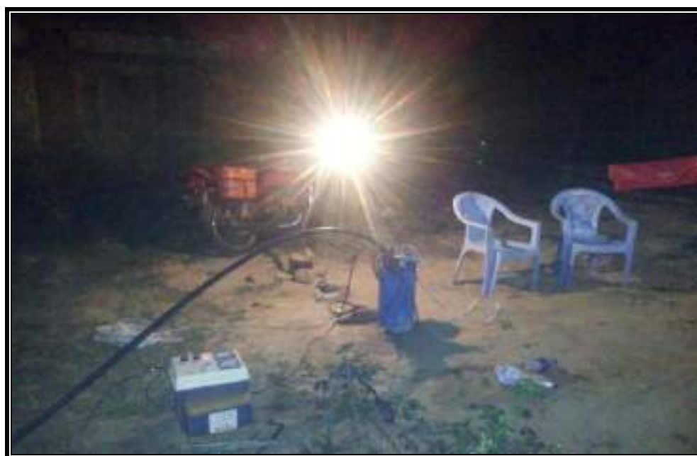
Photo 6: Pumping test assembly deployed in and around Jagannath OCP, Talcher coalfield, Odisha.
