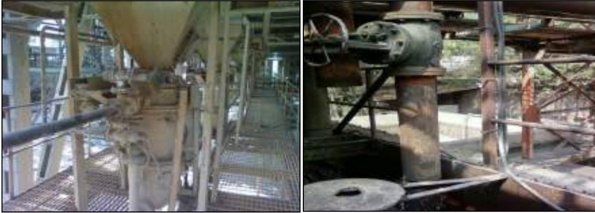
Figure 3.1 a) Collection of fly ash from ESP b) Collection of bottom ash from bottom ash hopper
