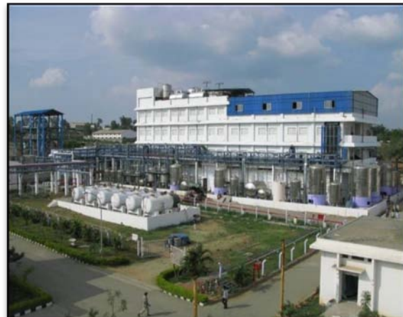
Photograph showing Main Production Block
