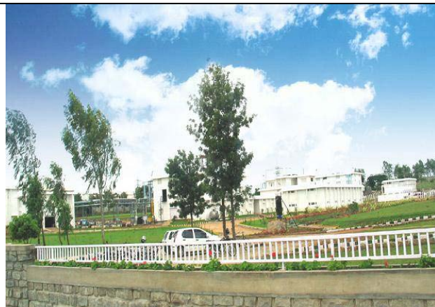
View of the Main Entrance of the Facility
