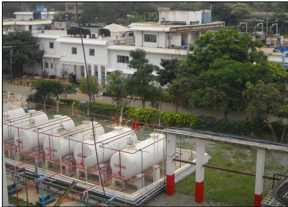
Figure 3-4: Solvent Storage Area
