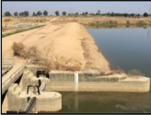
Raw water intake on Son River
