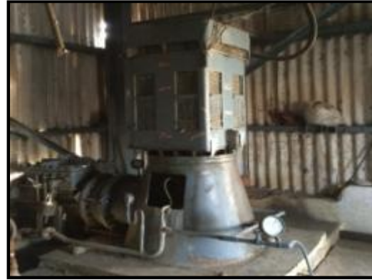
Raw water pump house
