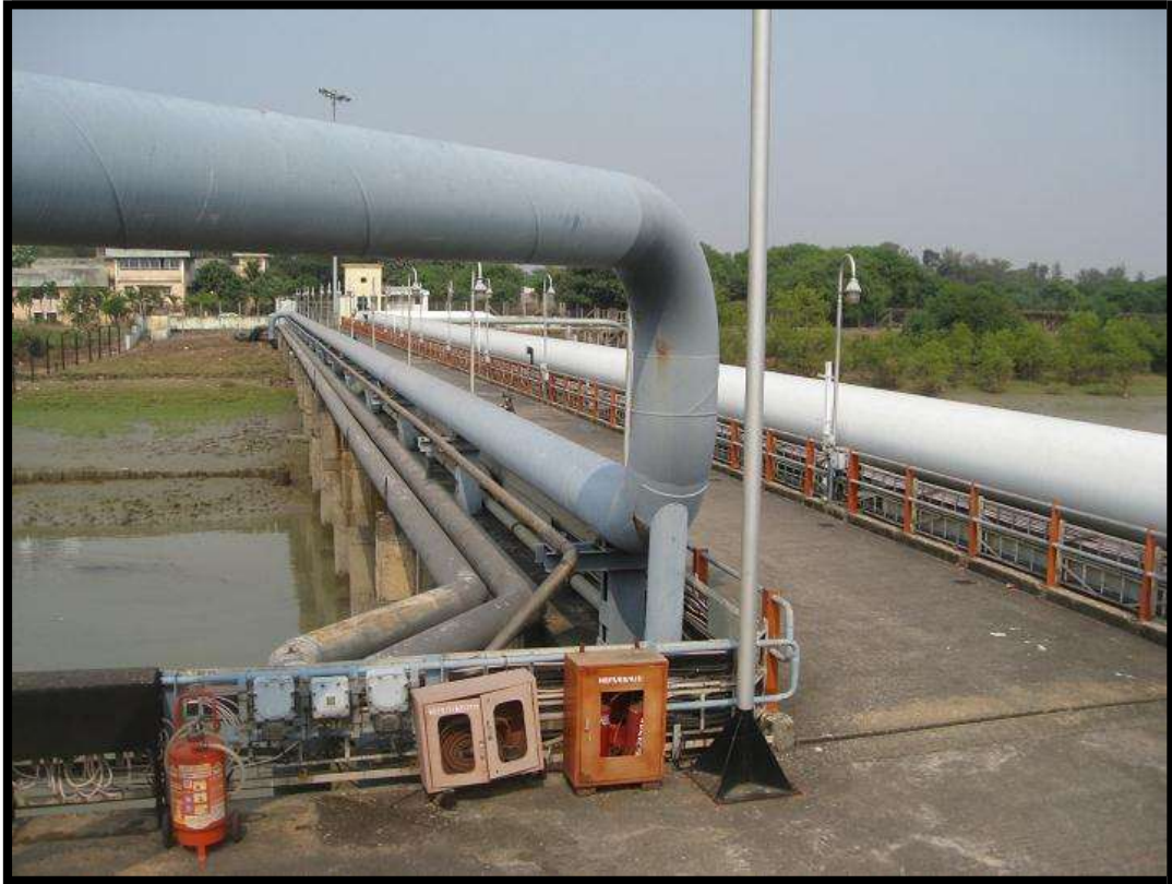
VIEW OF APPROACH TRESTLE
