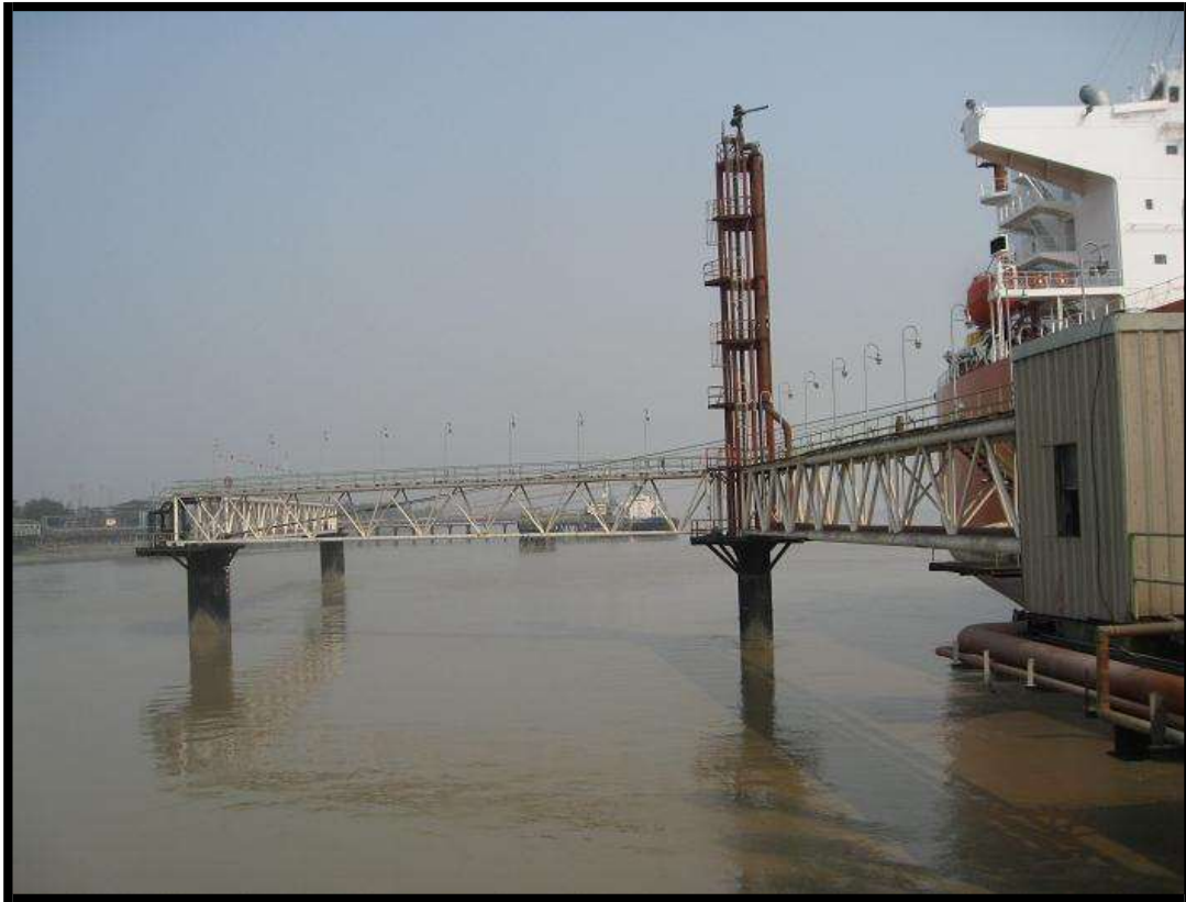
TOWER MONITOR & MOORING DOLPHINS
