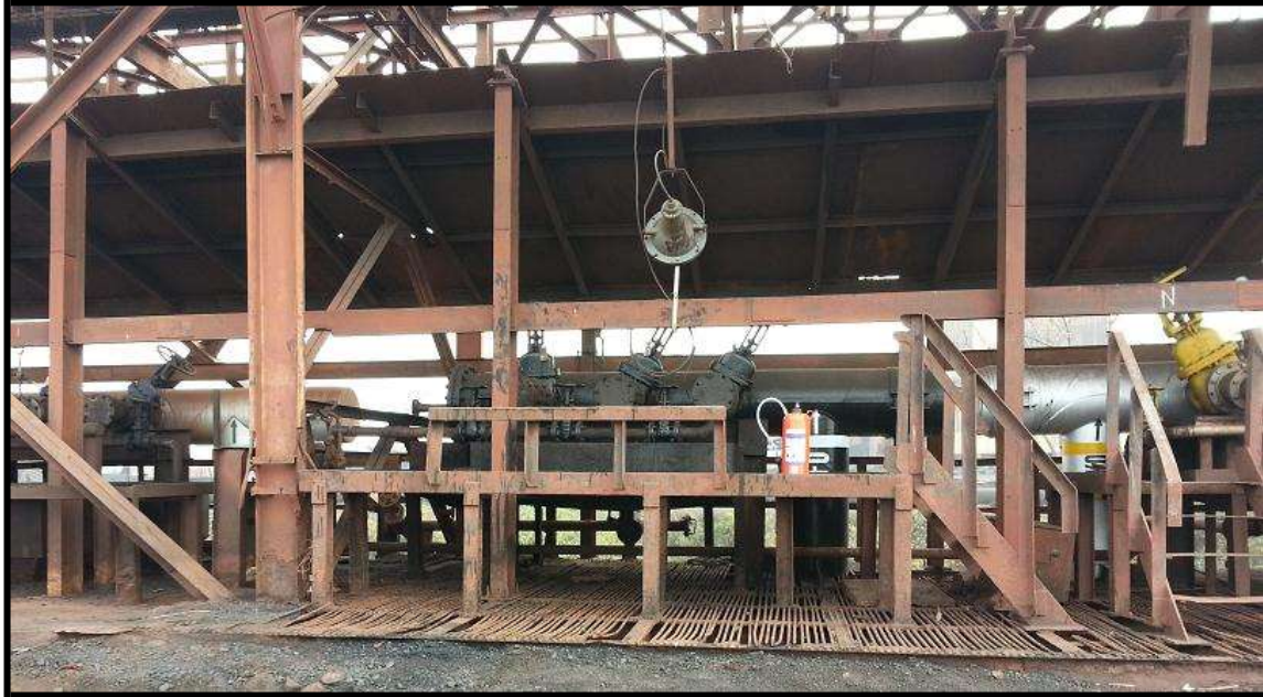
MANIFOLDS FOR BERTHS 2 & 3
