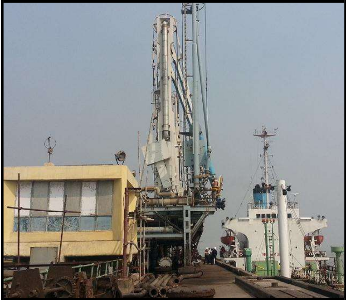
JETTY HEAD WITH UNLOADING ARMS & FLEXIBLE HOSES
