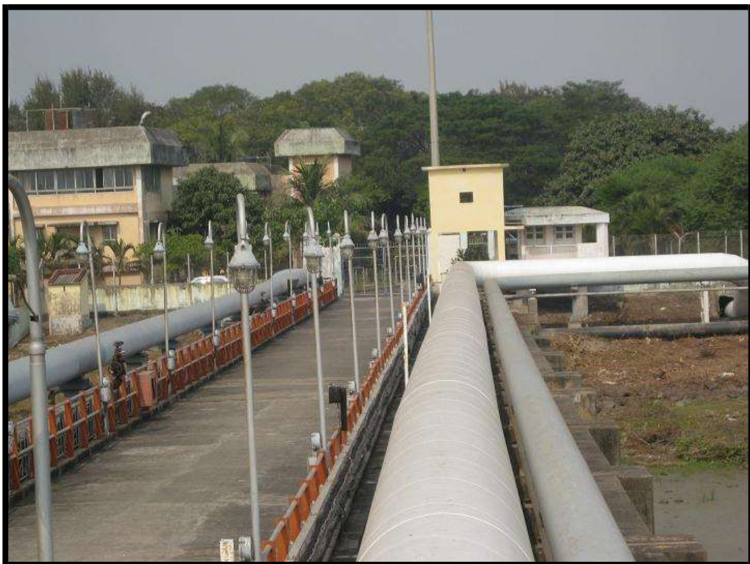
ANOTHER VIEW OF APPROACH TRESTLE
