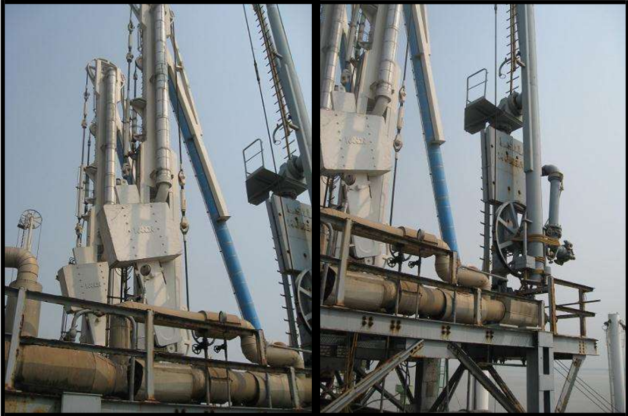
MARINE UNLOADING ARMS 2 X 10" AND 1 X 8"
