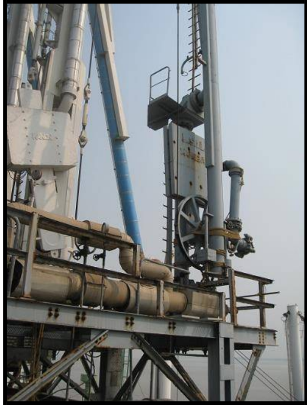
MARINE UNLOADING ARMS 2 X 10" AND 1 X 8"
