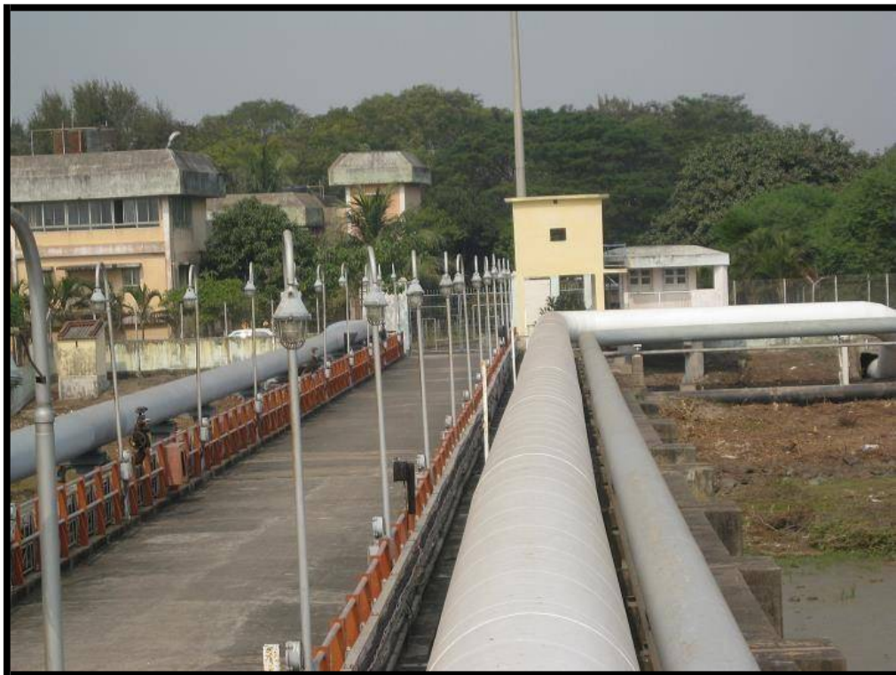
ANOTHER VIEW OF APPROACH TRESTLE
