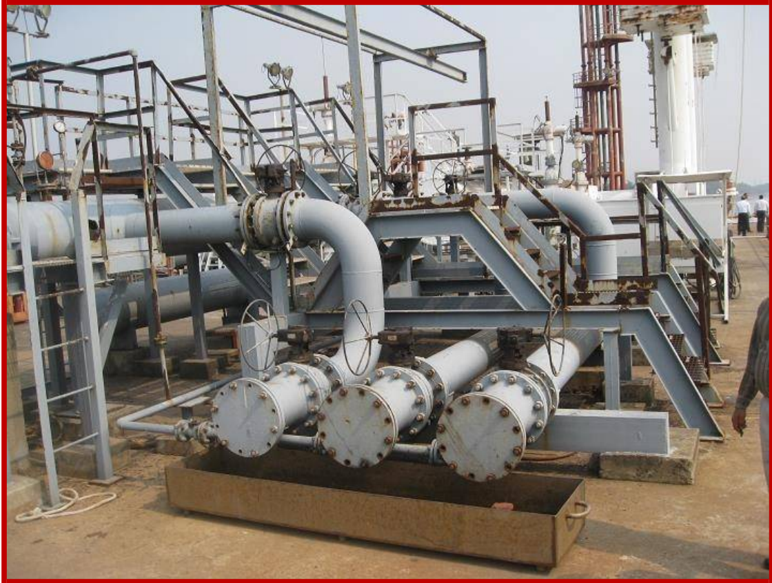
MANIFOLDS FOR FLEXIBLE HOSE CONNECTION
