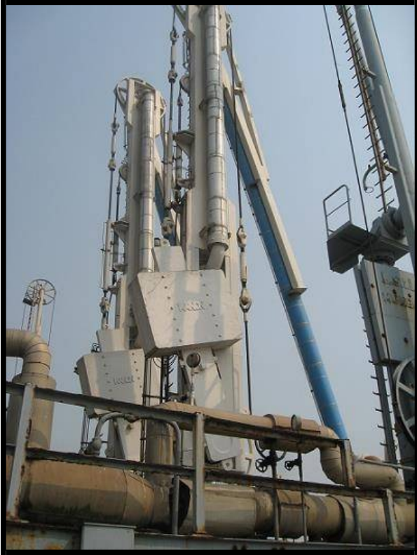
MARINE UNLOADING ARMS 2 X 10" AND 1 X 8"
