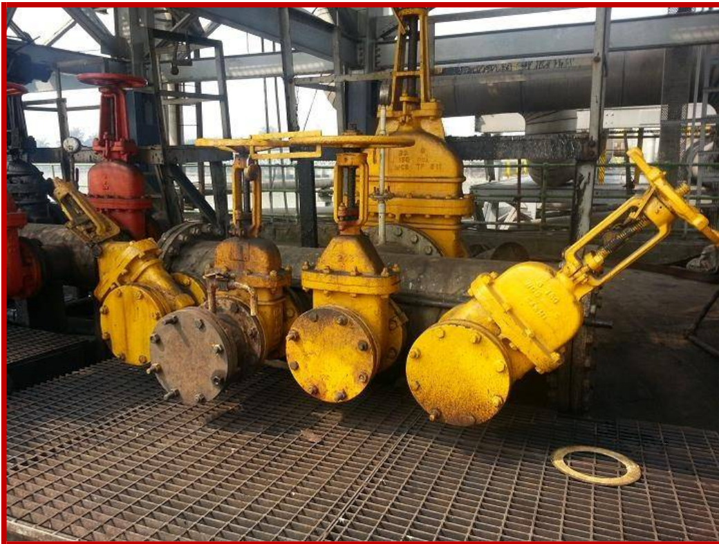
MANIFOLDS FOR FLEXIBLE HOSE CONNECTIONS
