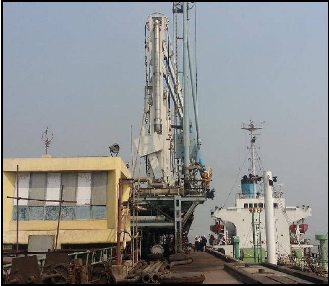
JETTY HEAD WITH UNLOADING ARMS & FLEXIBLE HOSES
