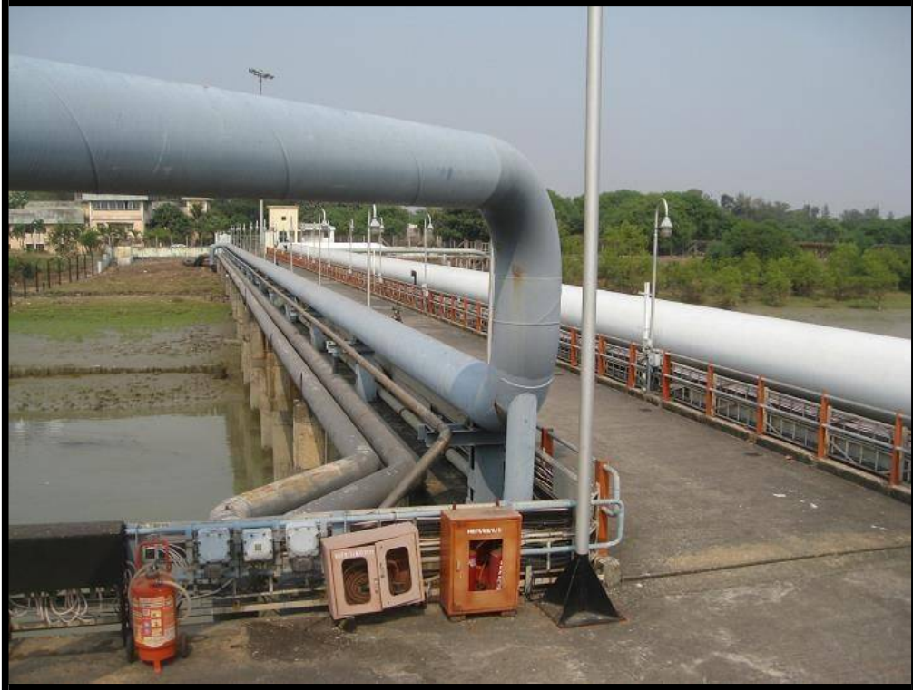
VIEW OF APPROACH TRESTLE
