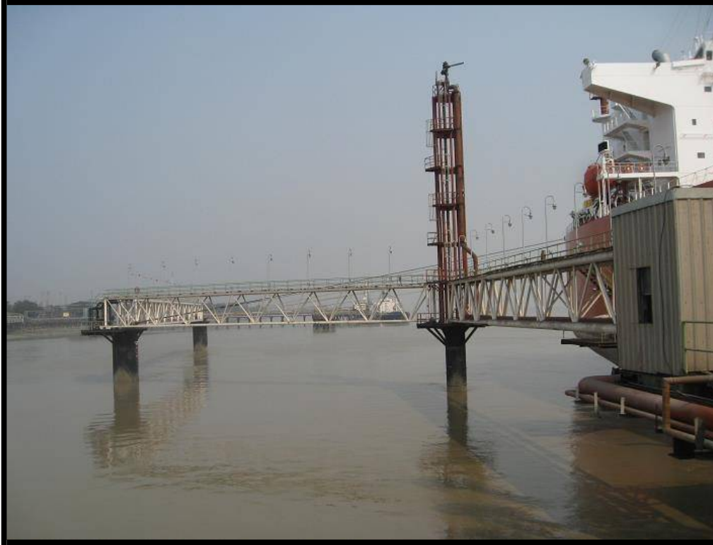
TOWER MONITOR & MOORING DOLPHINS
