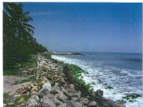
Plate 4: Seawall as HTL along seacoast
