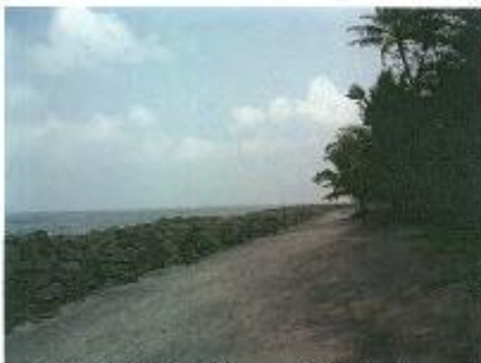
Plate 3: HTL getting modified due to slumping seawalls
