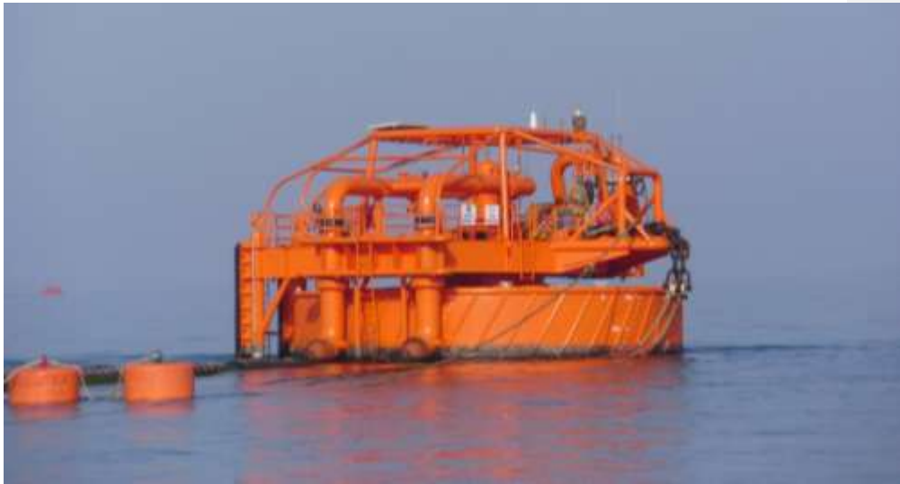
Figure 4 Single Point Mooring of BORL
