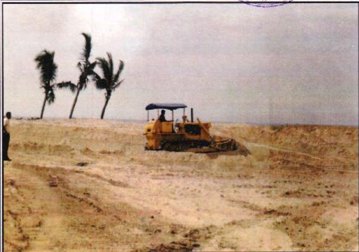
AREA REFILLED AFTER DREDGING BY IRE LTD IN ADJACENT BLOCK
