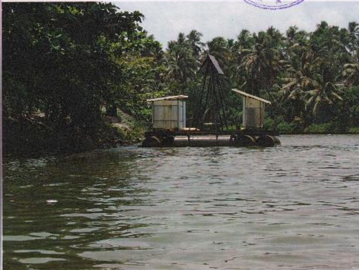
TOYO PUMP AND PONTOON ASSEMBLY IN CANAL
