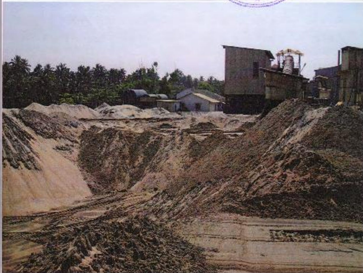
HEAP OF RAW SAND IN M.S. PLANT
