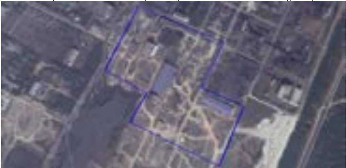
Fig. 11.6 - Google Earth Image of 21st Dec., 2017 of Site of COB-5 inside Visakhapatnam Steel Plant(Battery Erection Works in Progress)
