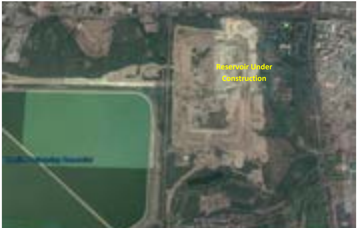
Fig. 11.7 : Google Earth Image of 13th April, 2018 of Site of New Water Reservoir
