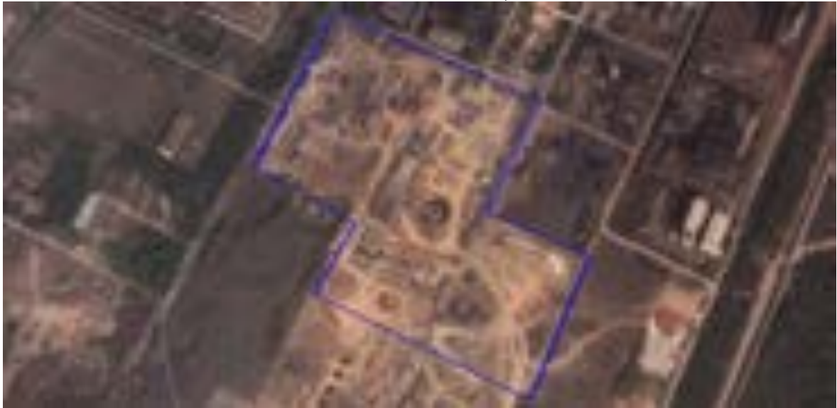
Fig. 11.5 : Google Earth Image of 15th Dec., 2016 of Site of COB-5 inside Visakhapatnam Steel Plant(Coal Stocks Almost Completely Cleared. Structural Erection Works at Site Started)
