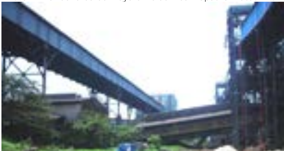
Photo 11.10: Covered Conveyors inside Visakhapatnam Steel Plant
