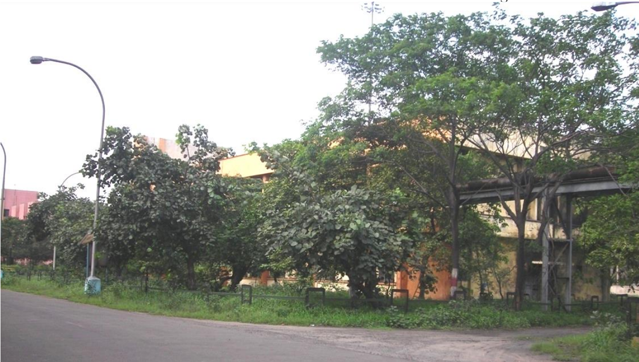
Photo 11.14: Tree Plantation around Office Building inside VSP
