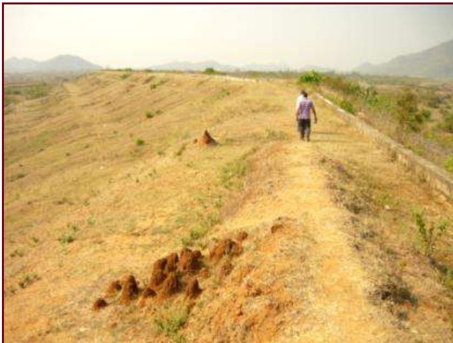
PHOTOPLATE-2.6. EMBANKMENT OF JANJHAVATI PROJECT
