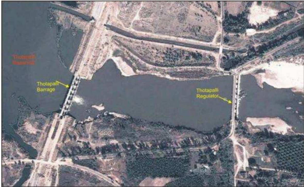
FIGURE-2.4 GOOGLE IMAGE SHOWING TOTAPALLI BARRAGE AND REGULATOR
