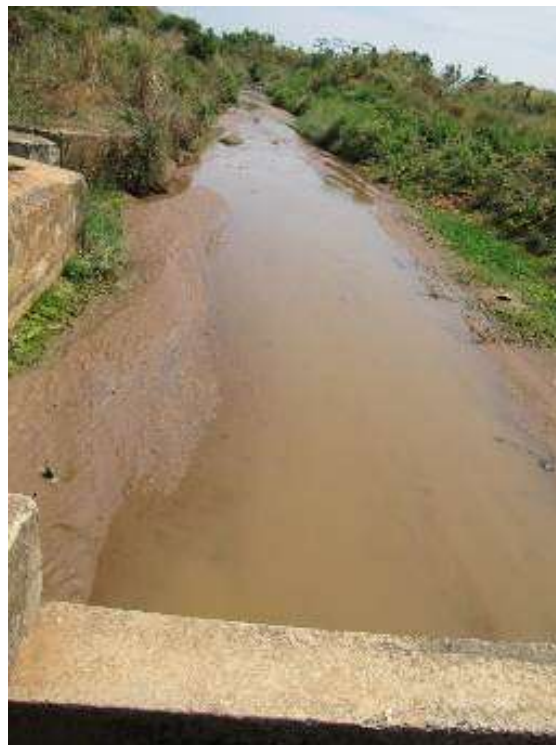
FIGURE-12 THE RUBBER DAM AND THE FLOW DOWNWARDS OF THE JHANJAVATHI RIVER AND THE CANAL
