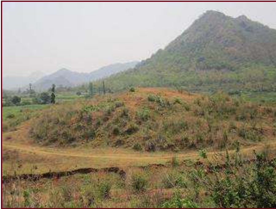
PHOTOPLATE-2.8. EMBANKMENT OF VAKAKABADI GEDDA PROJECT (UNDER CONSTRUCTION)
