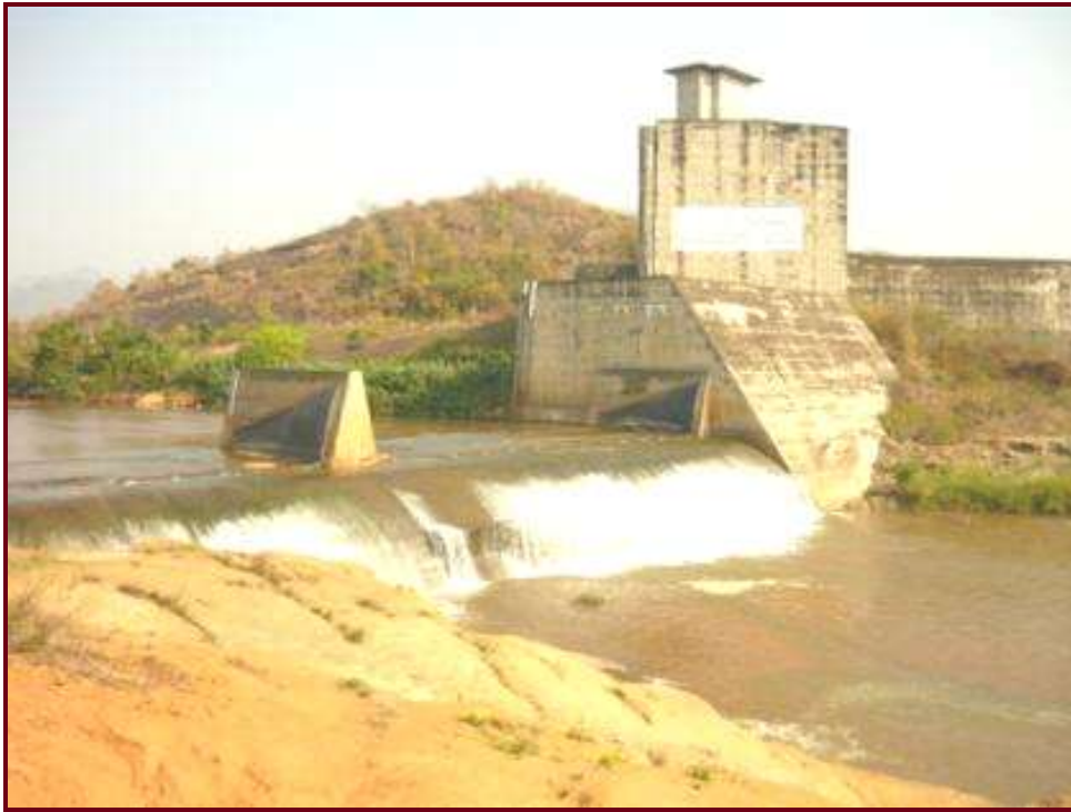
PHOTOPLATE-2.5. JANJHAVATI PROJECT (RUBBER DAM)
