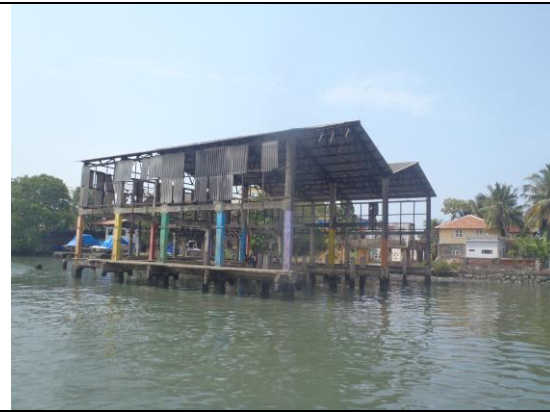
Plate 2. Existing workshop and boat yard
