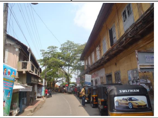
Plate 4. The existing township and human settlement along the western margin of the project site.
