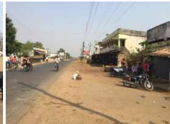
Road section in Balaghat
