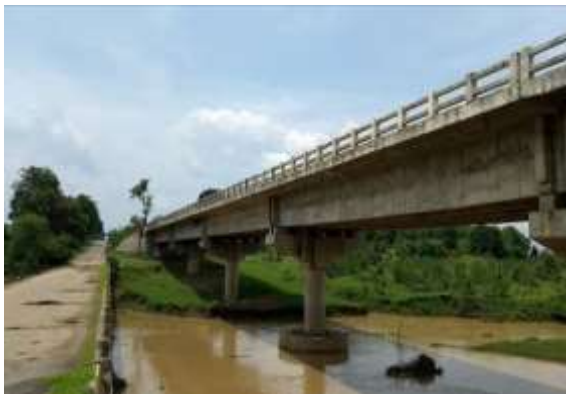
Bridge on Ghisari River at Existing Chainage 19+901
