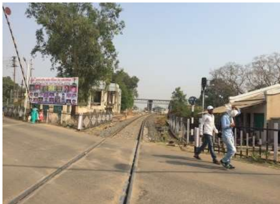
Level crossing at Km 2+431
