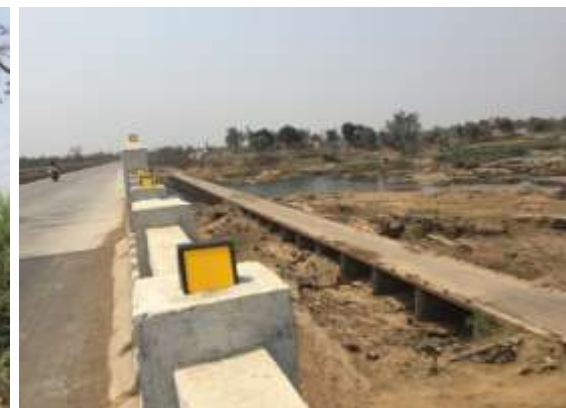
Bagh River Bridge on Border at km 24+359
