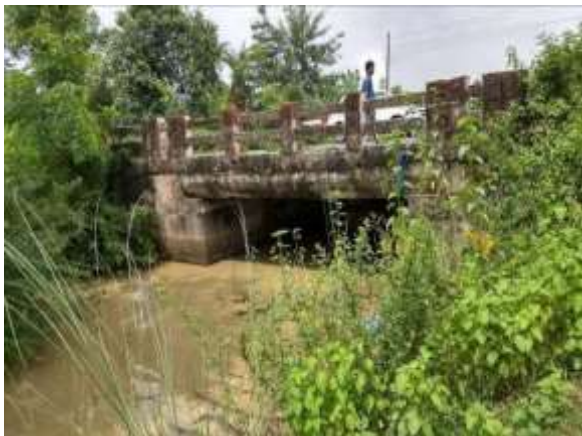
Bridge at Existing Ch.28+498
