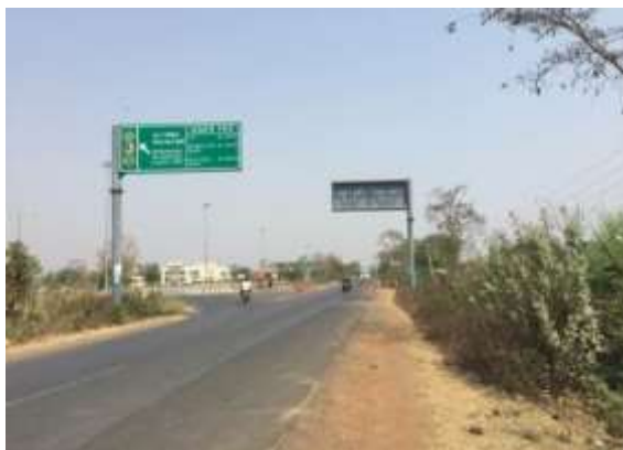
Check post at Km 21+600
