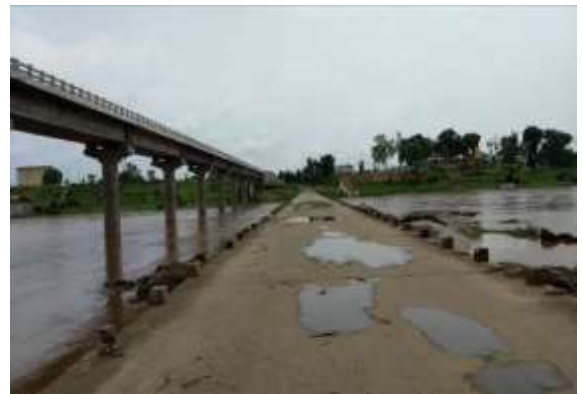
Bridge on Bhagh River at Existing Ch.24+359
