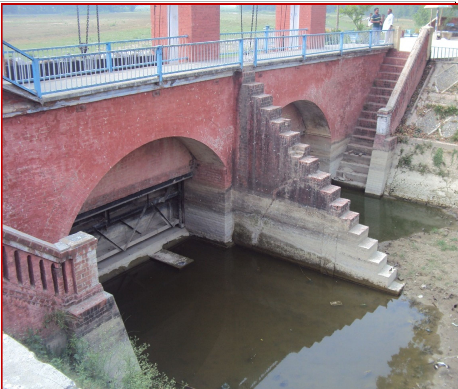
View of Head Regulator of Kosi Canal
