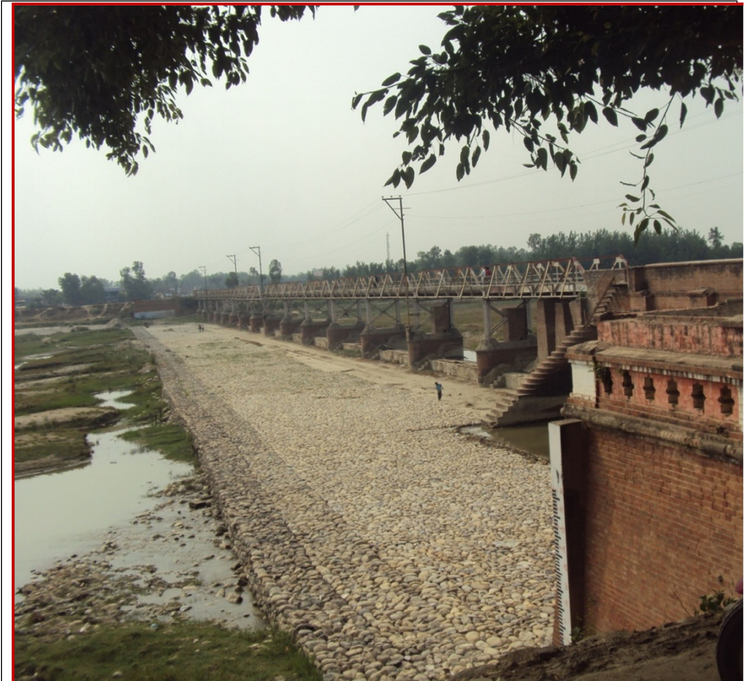
Downstream view of Lalpur Weir
