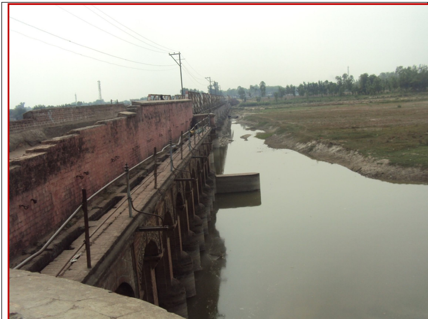
Upstream view of Lalpur Weir
