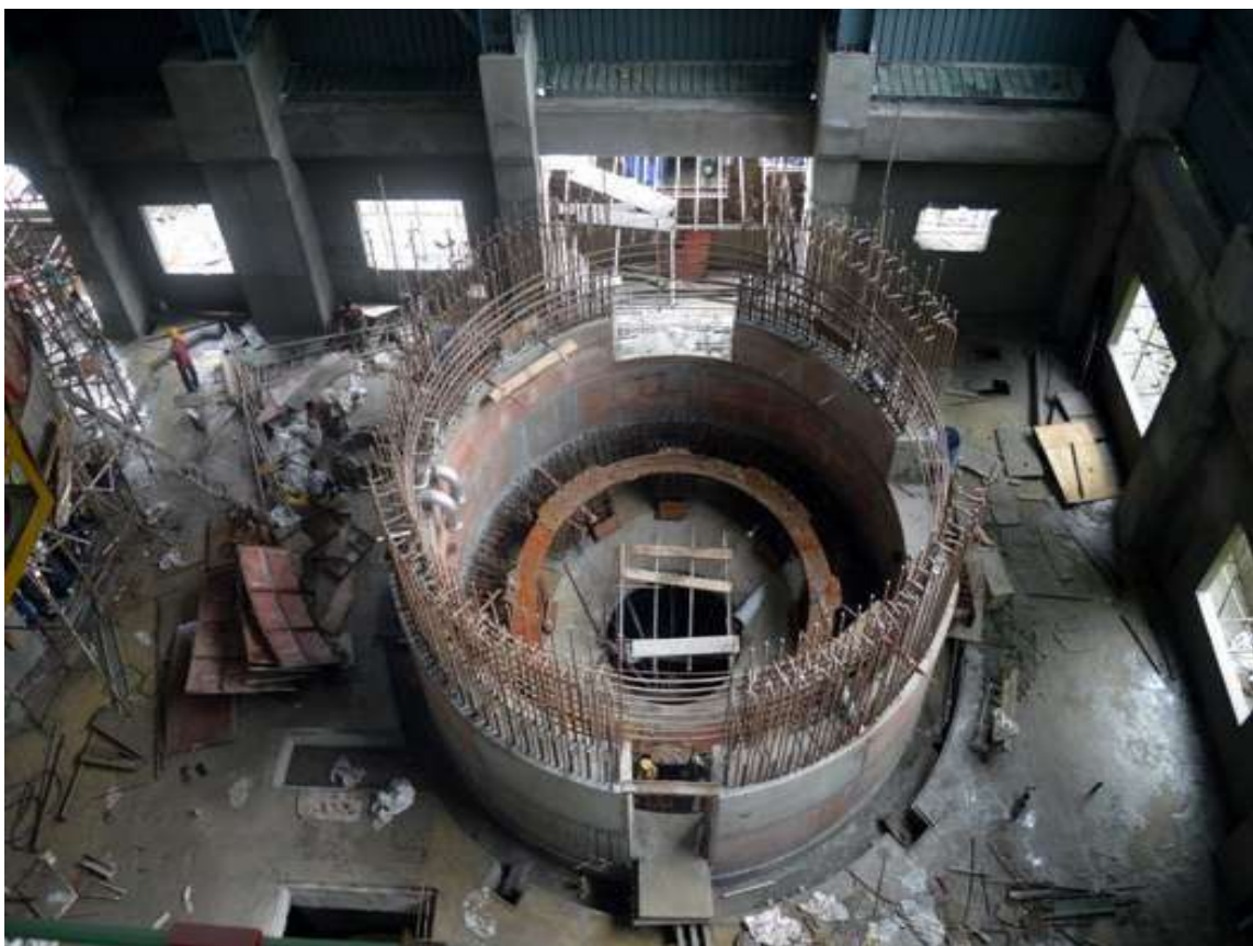
Figure 8: Concreting of Generator Barrel Unit-2
