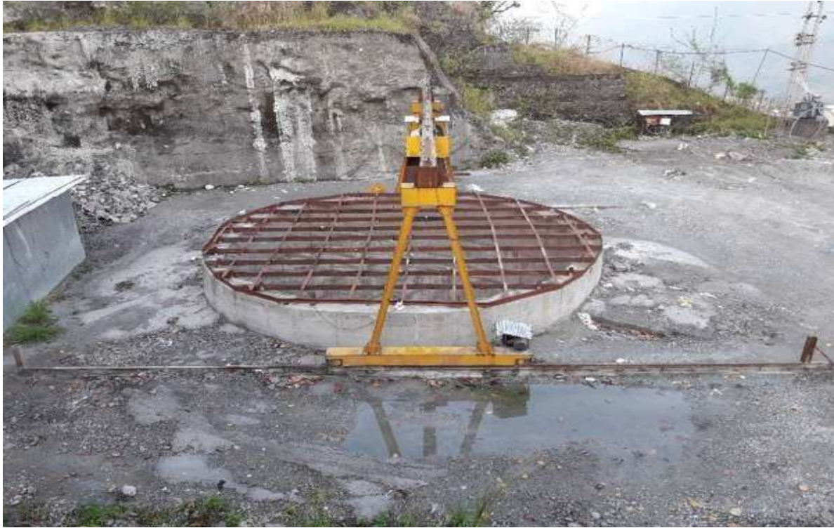
Figure 5: Surge Shaft Lining
