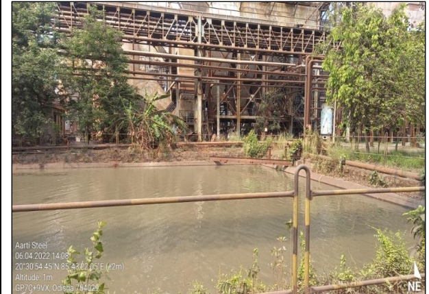
WASTE WATER SUMP
