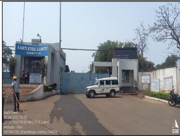
MAIN ENTRY GATE
