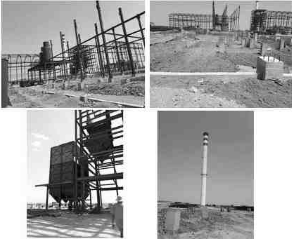
Existing Industry construction photographs
