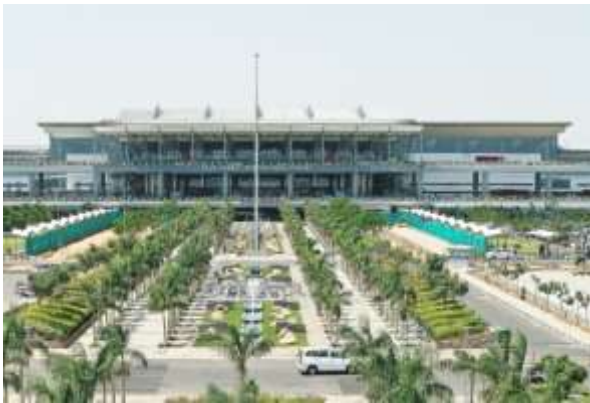
RGIA Passenger Terminal Building
