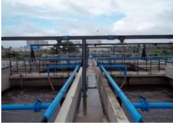
Sewage Treatment Plant
