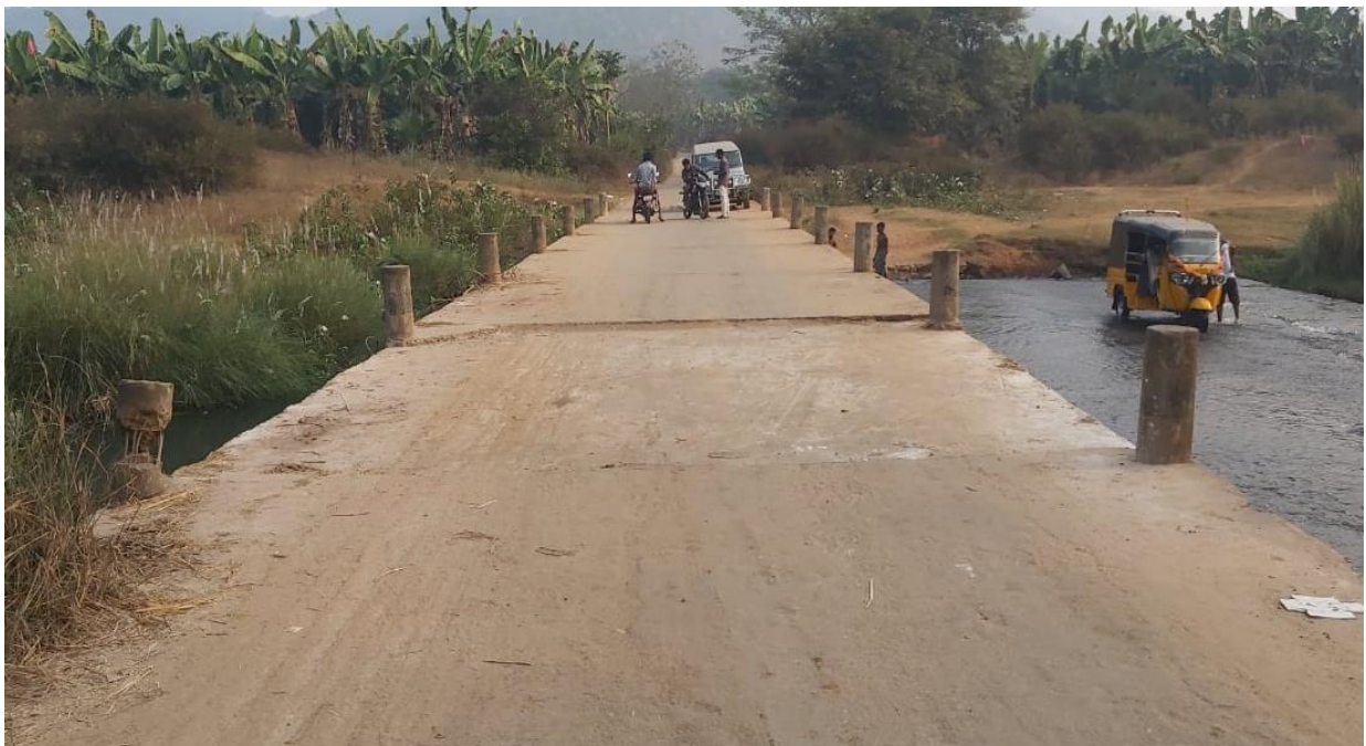
Low Level Causeway 6.3 km Downstream of Lower Dam (Near Dandigam)
