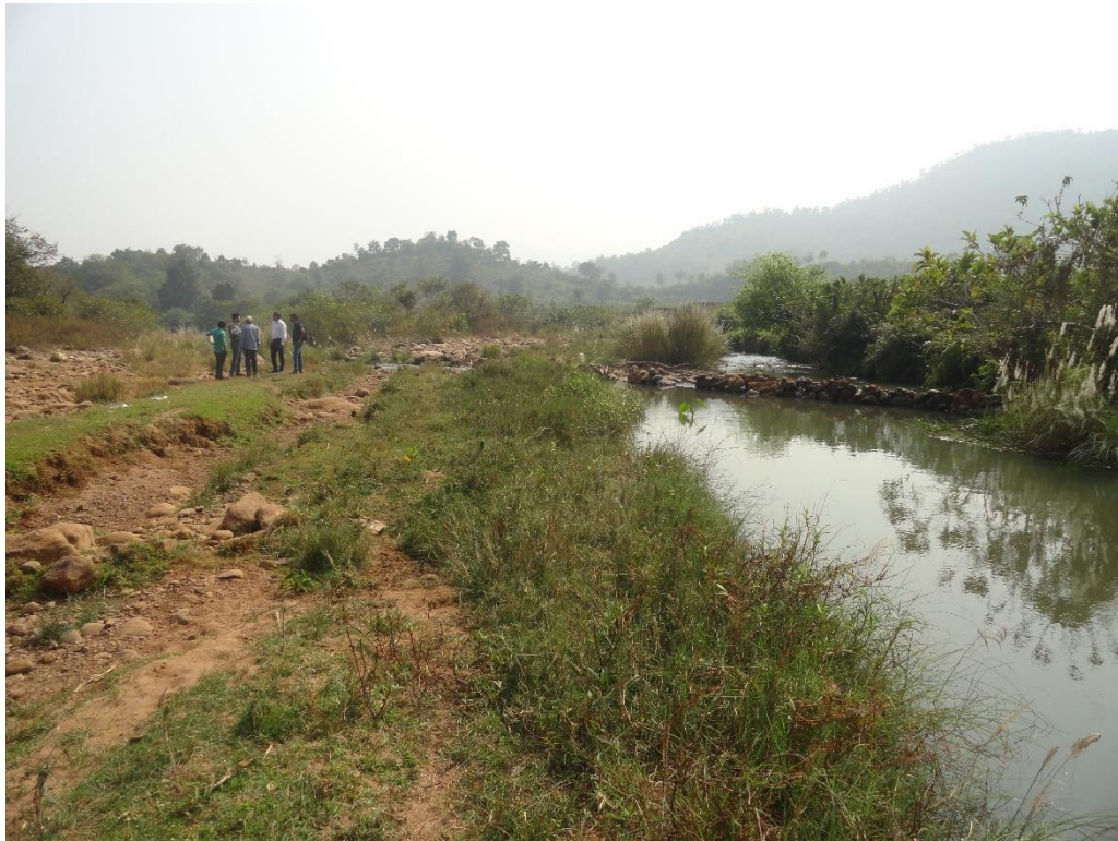
Lower Dam Site
