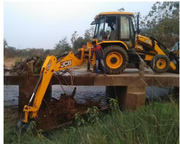
Site Clearance Works
