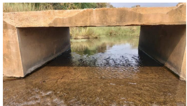
Gauging Station (After Site Clearance)
