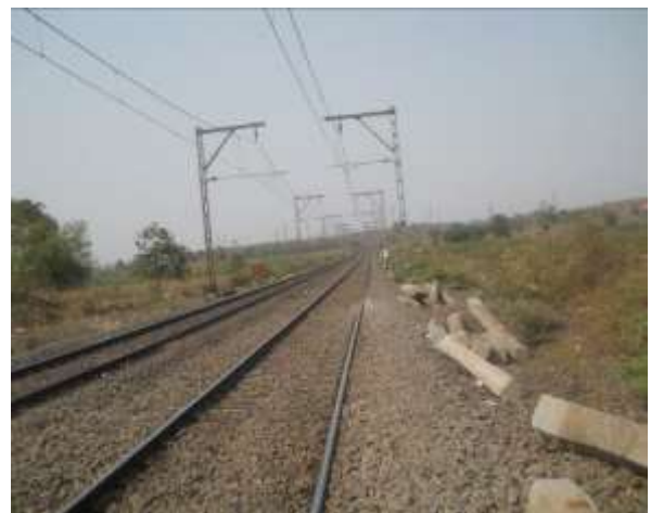
Crossing with Railway line at km 47.940
