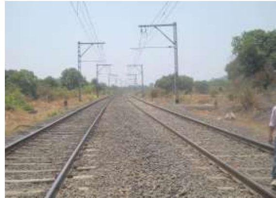
Crossing with Railway line at km 67.500
