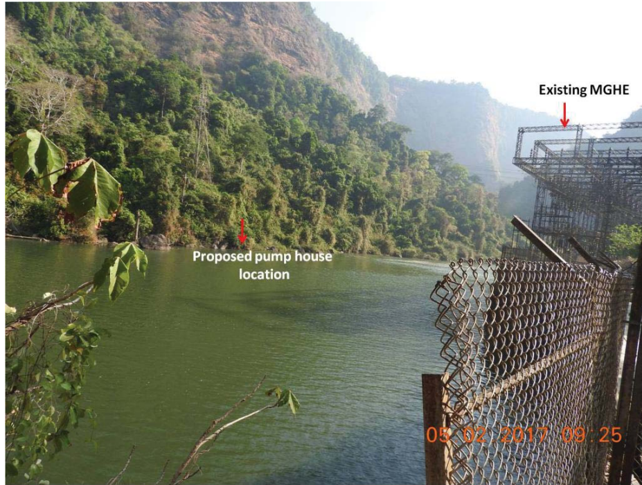
Fig - 2 Photograph showing pump house location
