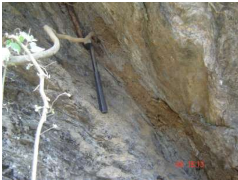
Photograph-4: Shear zone near Khuni Gad Bridge
