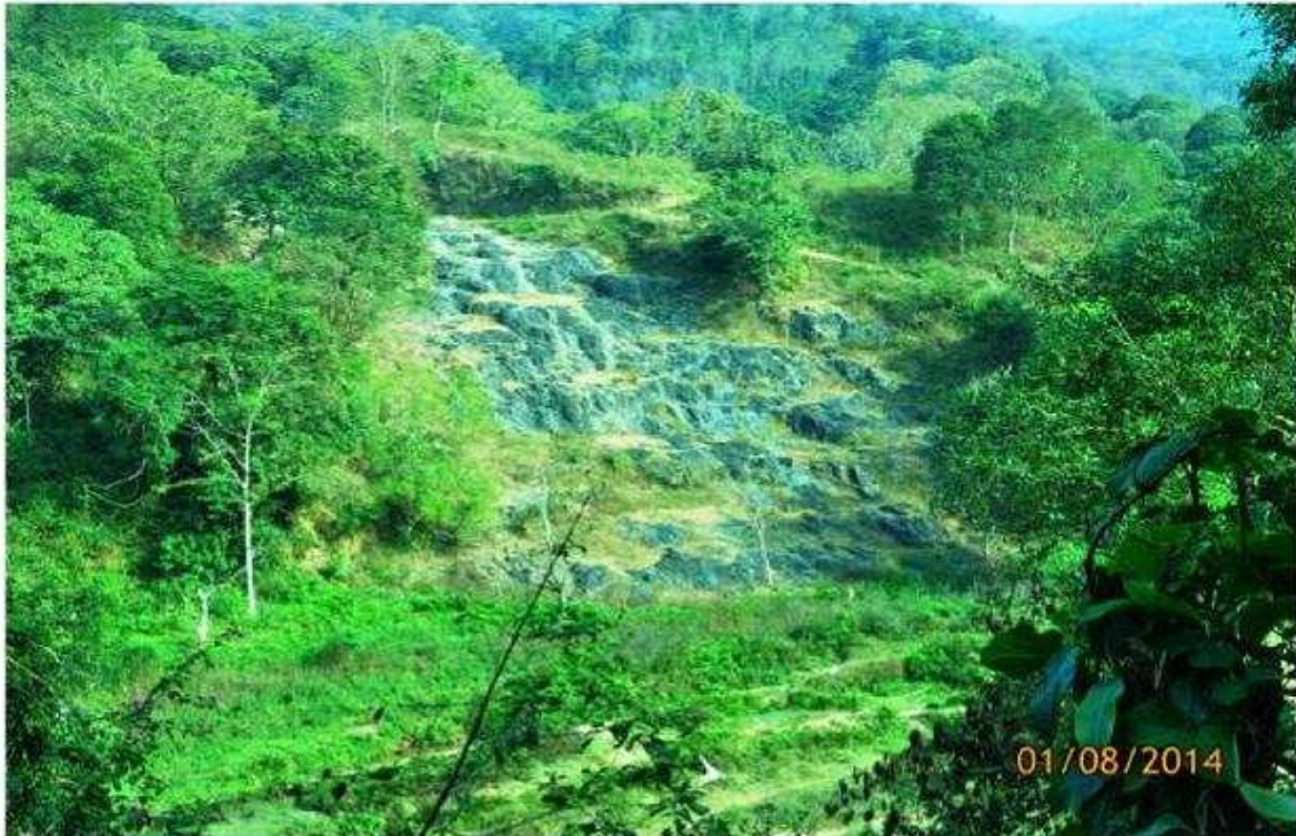
Partially completed blasting for foundation on Right flank of dam
