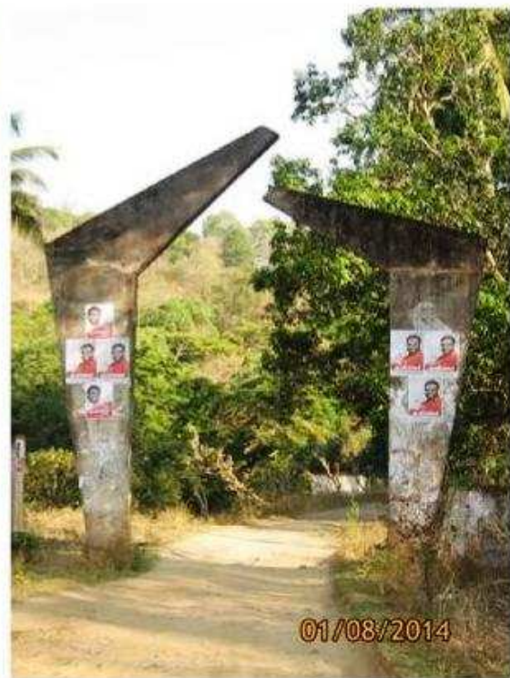
Entrance arch of AVIP dam site
