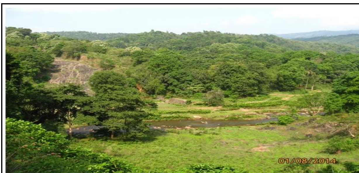
Right flank of dam & Siruvani river- View from left flank of dam
