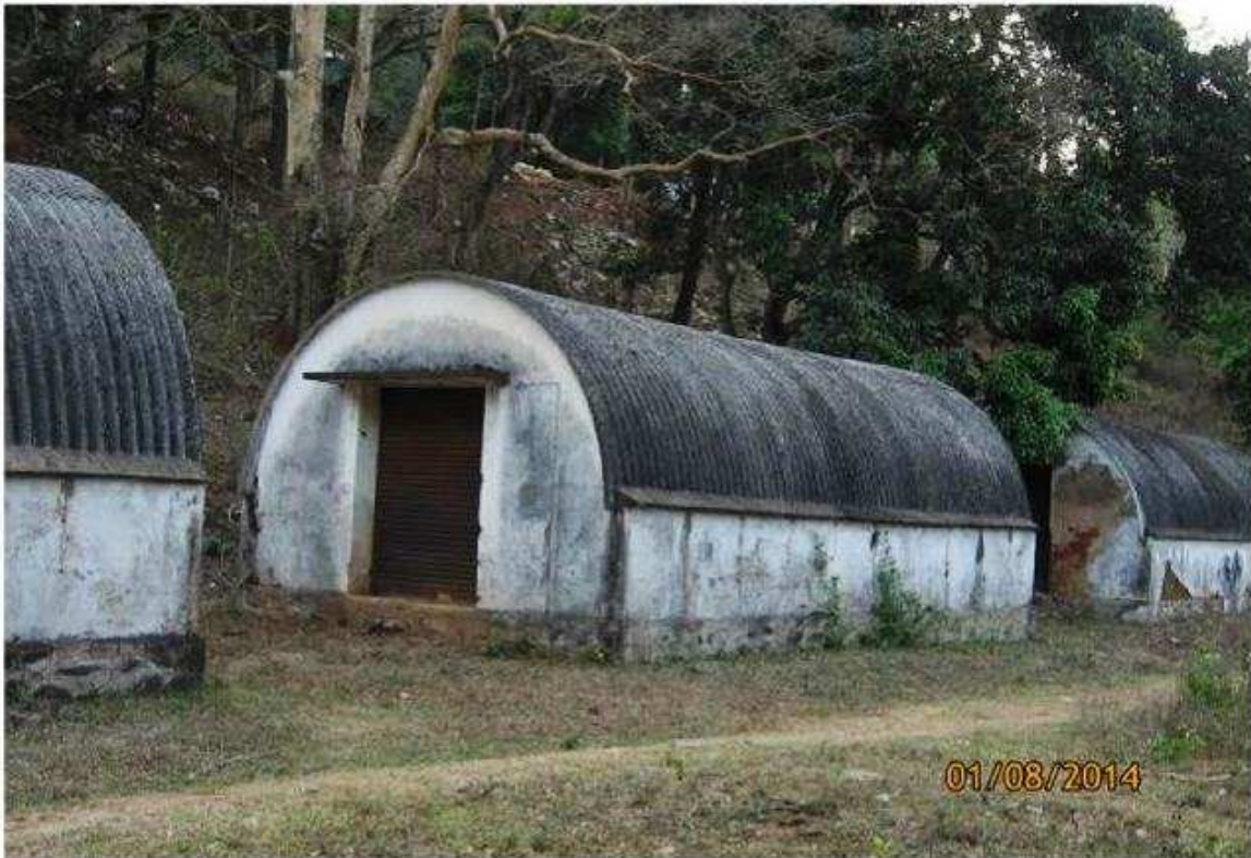
Stores at Chittur dam site
