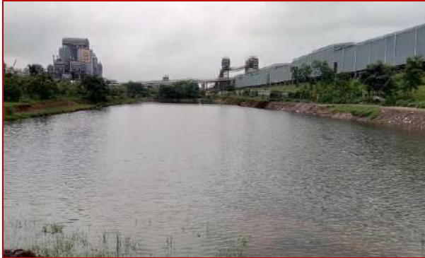
Rain Water Harvesting Sump at NE corner of the Plant
