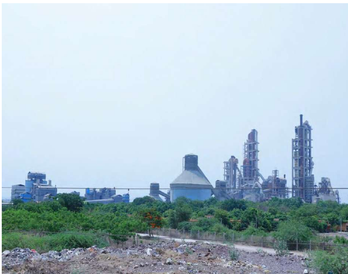
View of the Cement plant of M/s My Home Industries Ltd.
