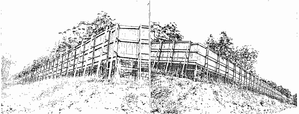
Wind Barrier Sheeting Outside view
