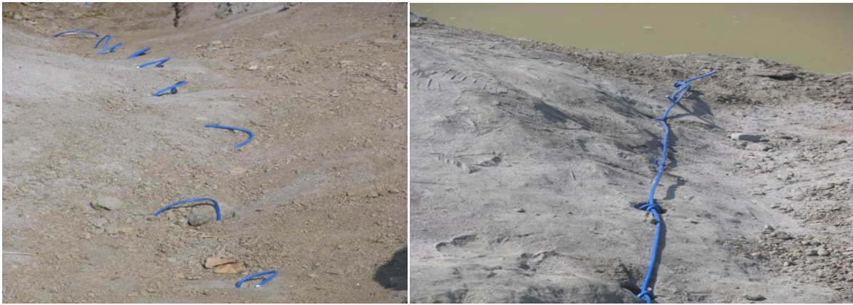
Figure 3.2.: Shot holes with low explosives connected with Detonating Cord (Trunk Line)
