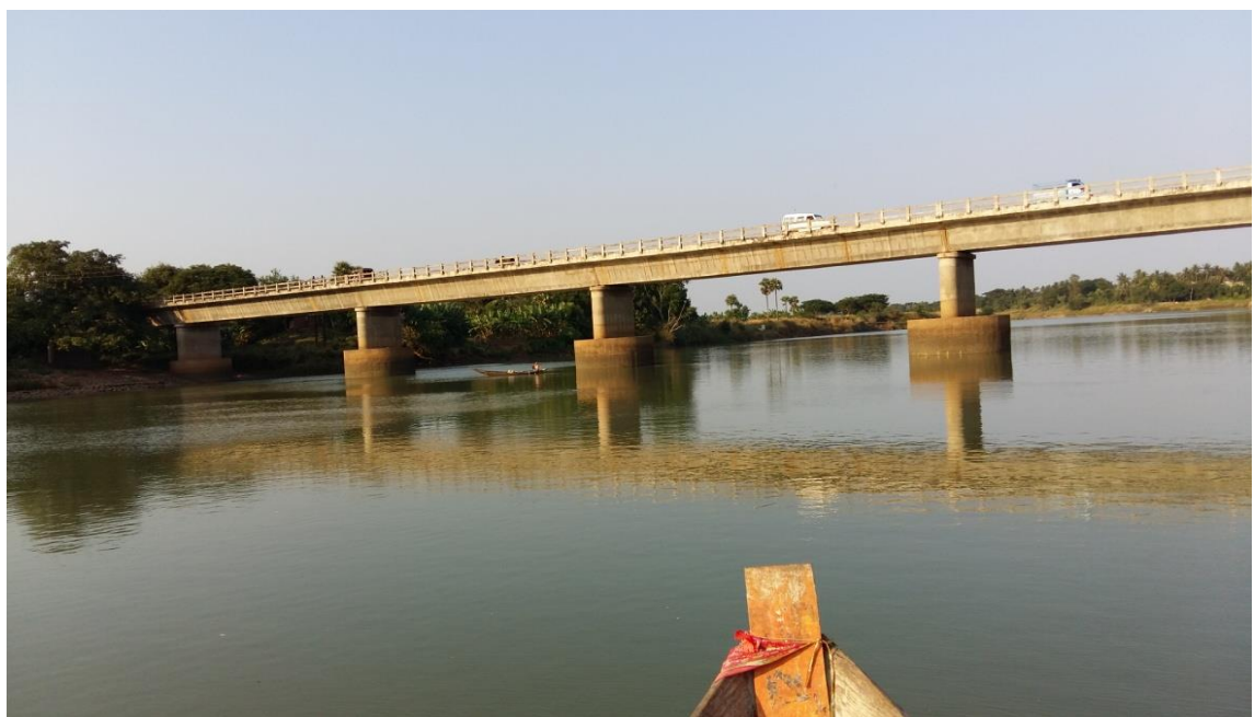
Figure-6: Manpur bridge (Up stream view)
