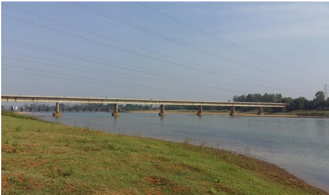
Figure-7: Jokadia barrage, bridge and powerlines (D/s view)
