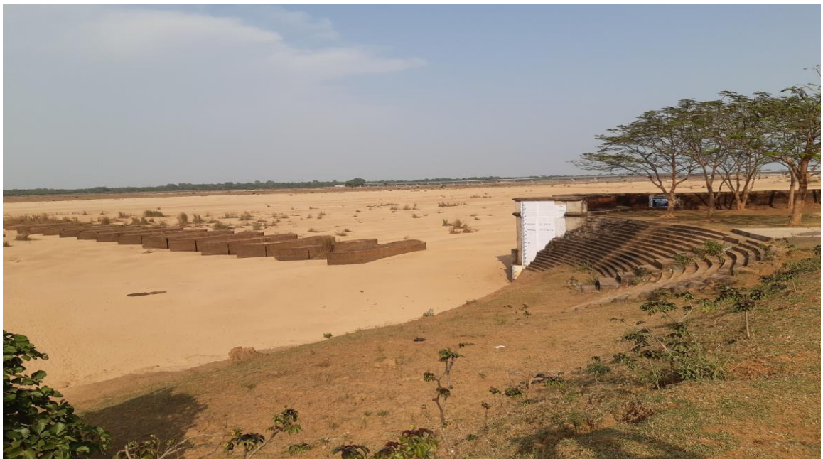
Figure-5: Defunct Jenapur weir (View from right bank)
