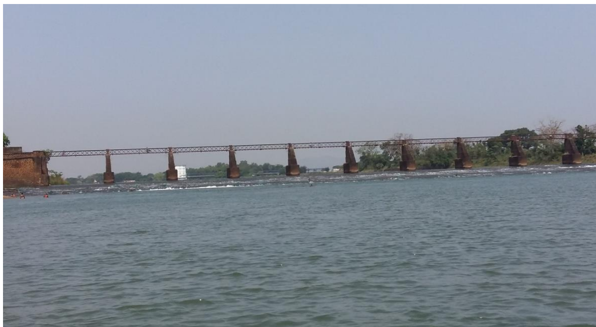
Figure-4 Jokadia Weir on River Kharsua (D/s view)
