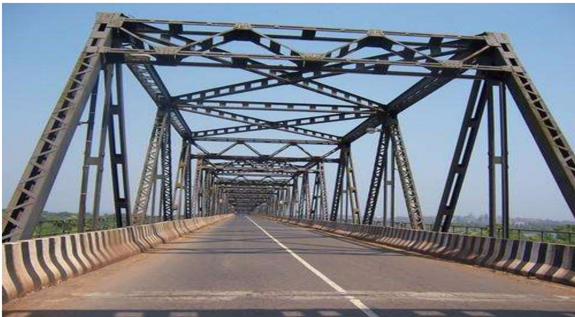
Fig 14: Typical Bridge on Zuari River
