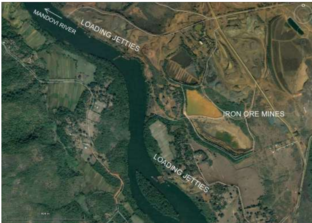
Fig. 10: Typical iron ore loading jetty locations along the banks of river Mandovi
