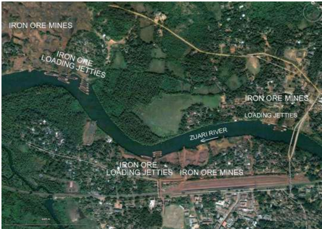
Fig. 9: Typical iron ore loading jetty locations along the banks of river Zuari
