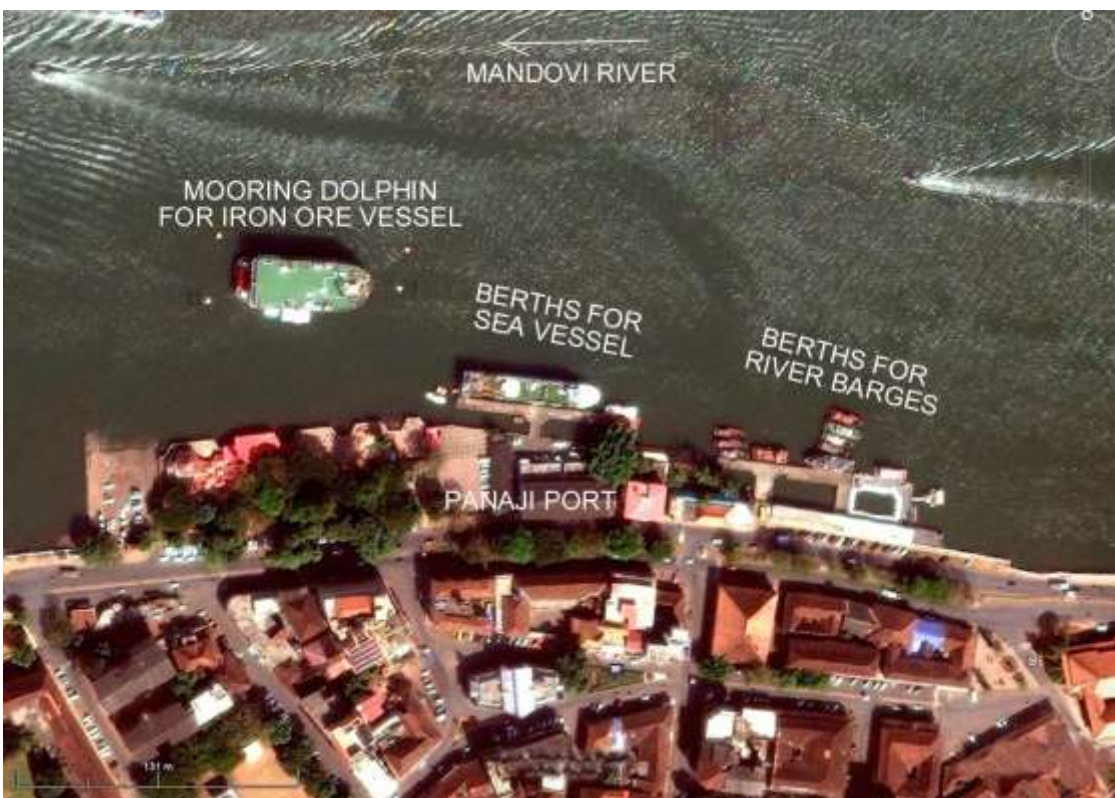
Fig 8: Panaji Port – Iron ore handling facilities
