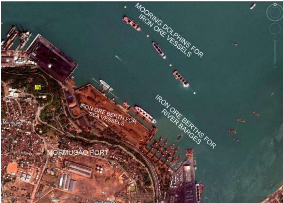
Fig. 7: Iron ore handling facilities at Mormugao port
