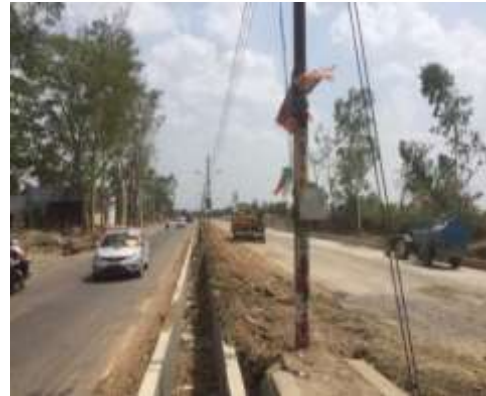
Under-construction 4 lane at Km 1+500
