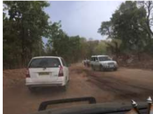
Under-construction road near km 20
