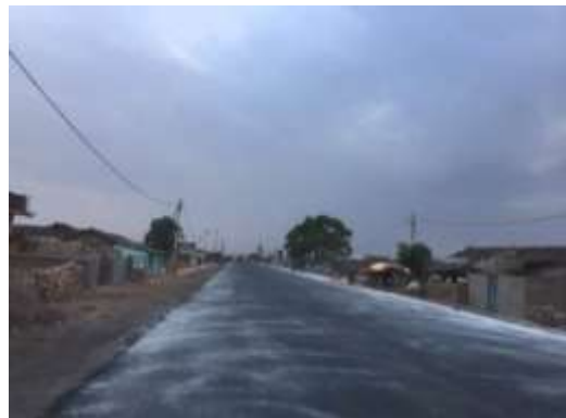
Recent done Bituminous work
