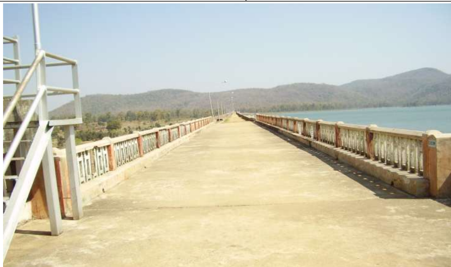
Right Flank of Earthen Dam
