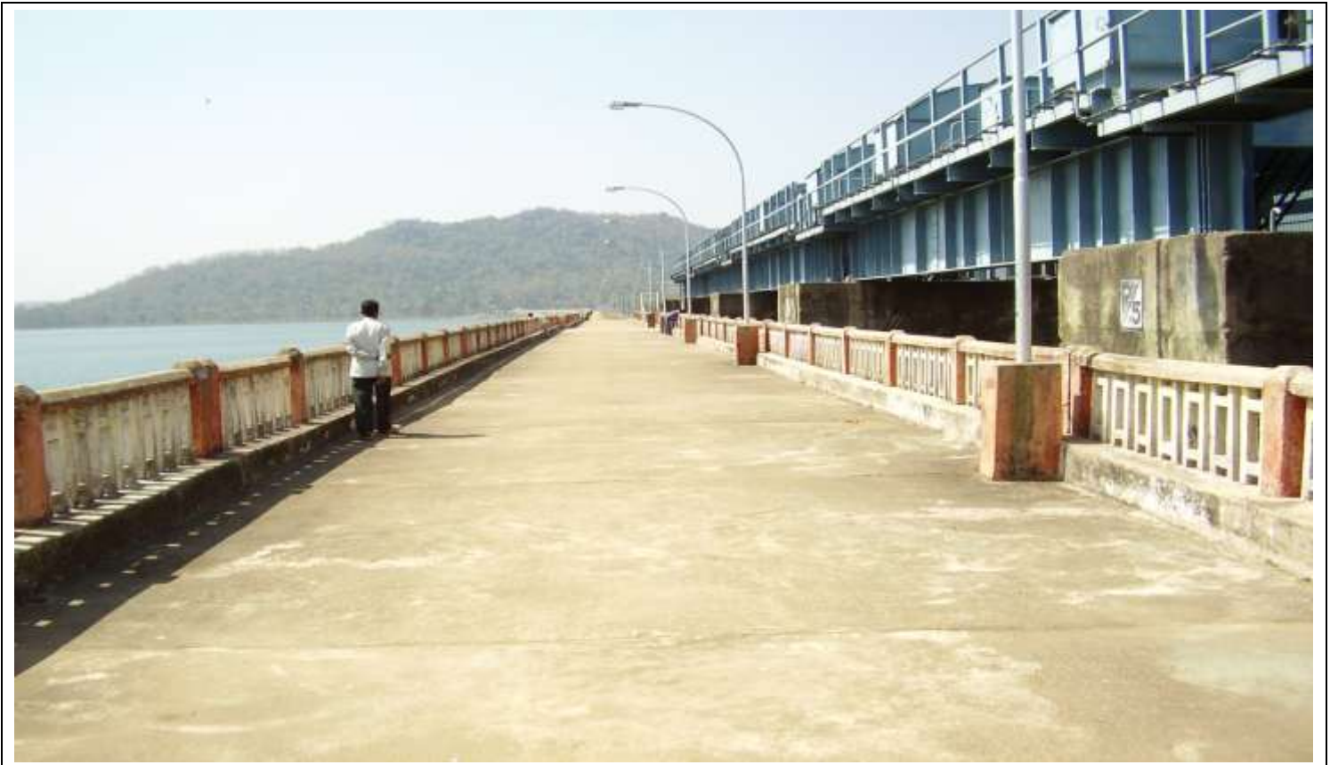
Left Flank of Earthen Dam
