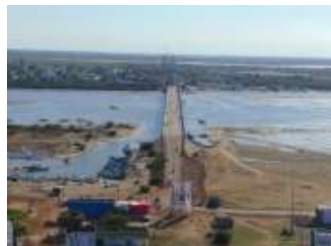
d. Aerial view of the existing Pulicat bridge
