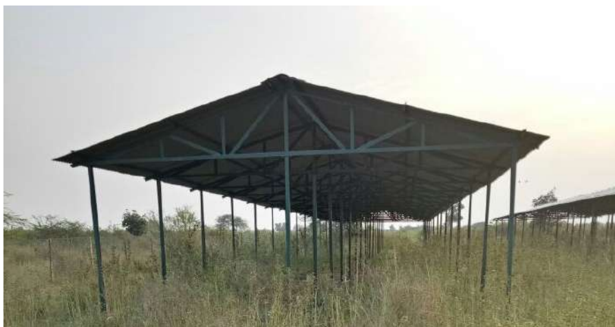
Figure 21 Construction 2 nos. of Cattle sheds
