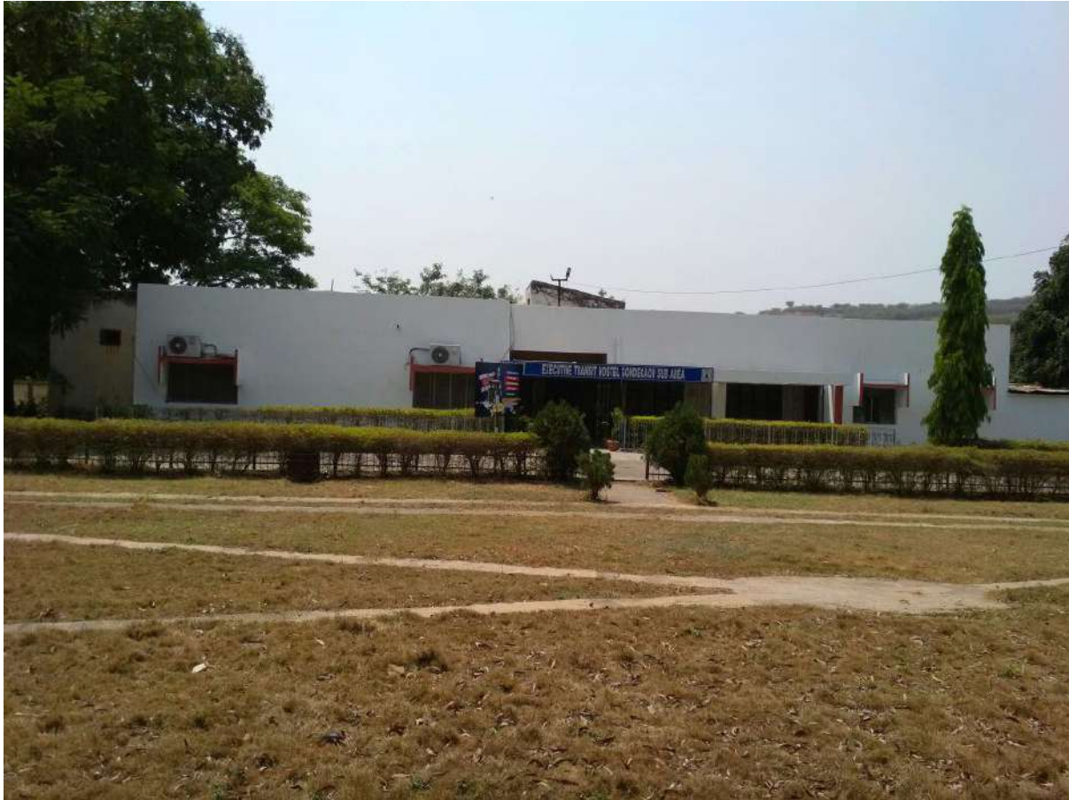
EXECUTIVE TRANSIT HOSTEL AT GONDEGAON
