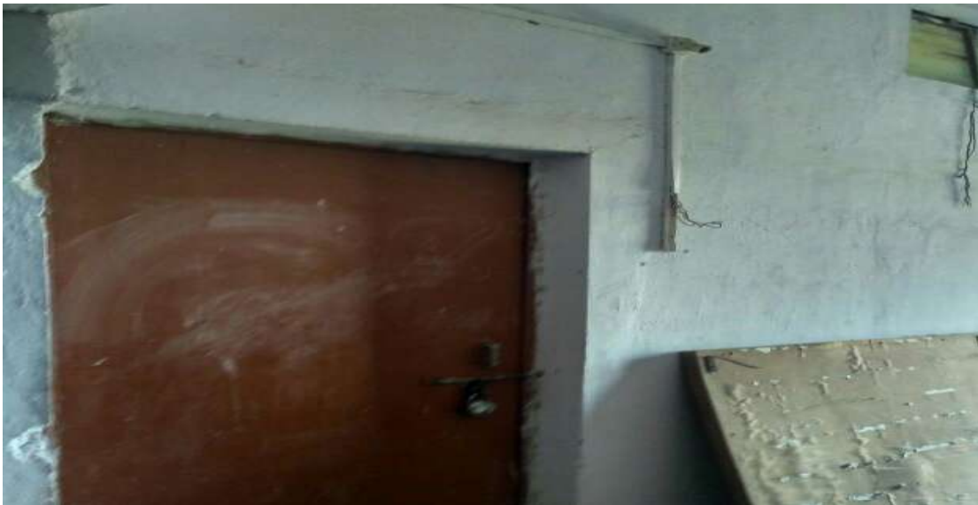
Figure 33 Construction of room at Porwal College Kamptee
