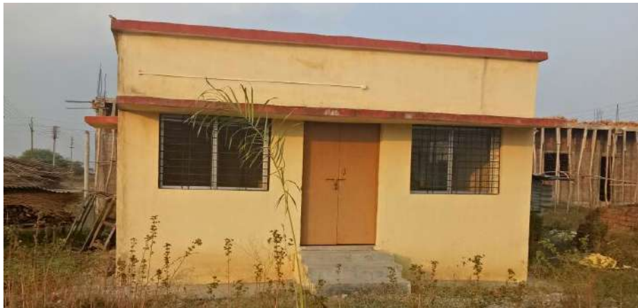
Figure 23 Construction of Aanganwadi
