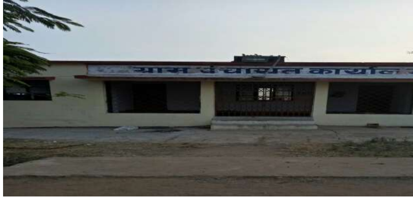
Figure 16 Gram Panchayat Office:
