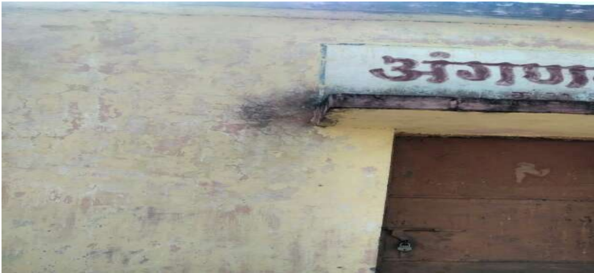
Figure 29 Construction of room for Anganwadi at Ghatrohna village
