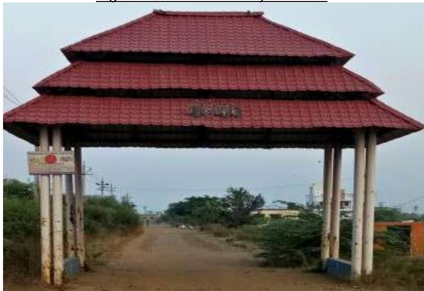
Figure 17 Construction of Entry gate at new Gondegaon Village
