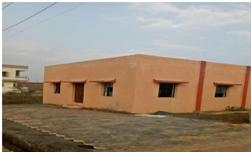
Figure 26 Construction of Post office & Bank Building under construction
