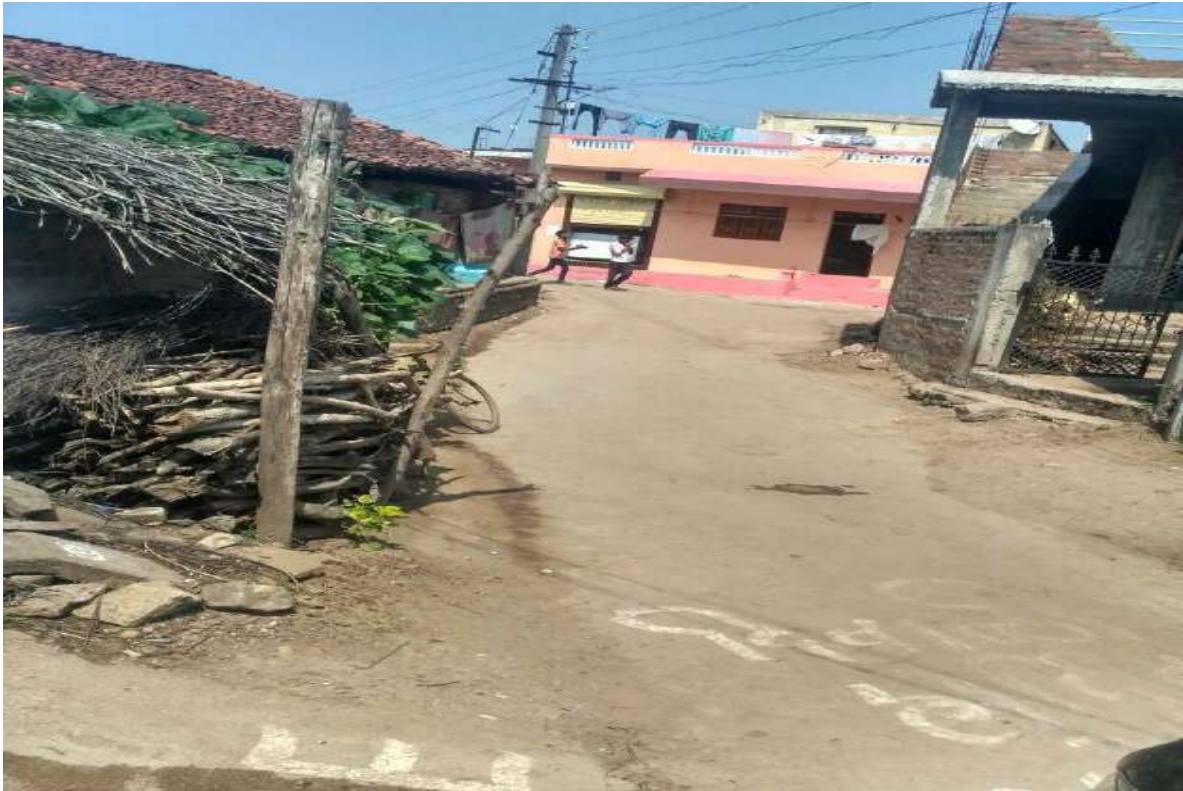
Figure 30 Repairing of damaged tar road from village Yesambha to Wagholi (length appr.3000 m).
