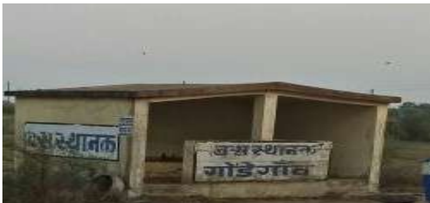
Figure 19 Construction of Bus Stoppage
