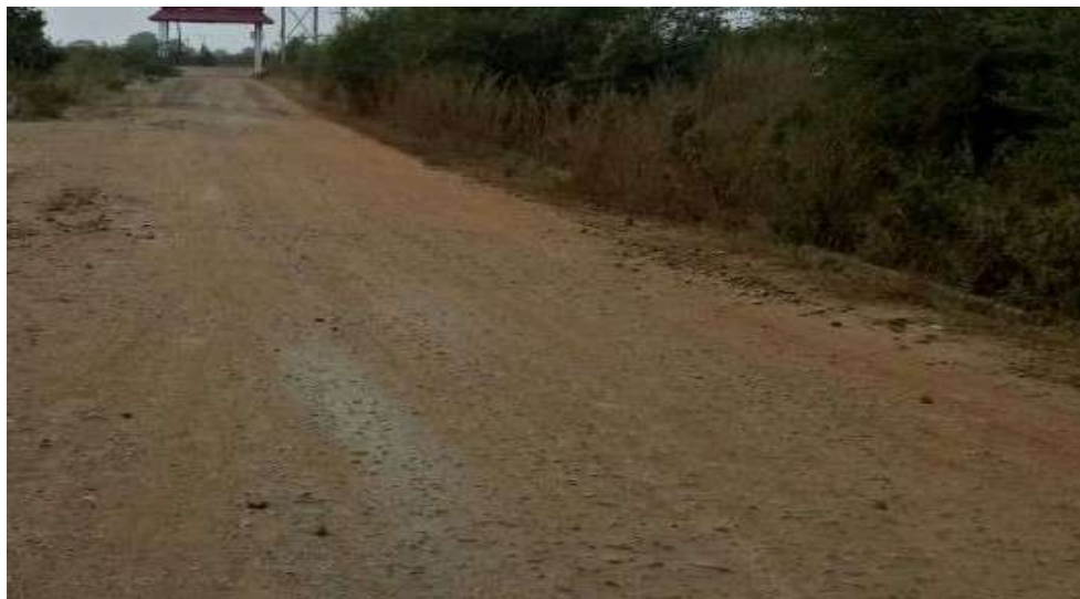
Figure 25 Construction of WBM Road
