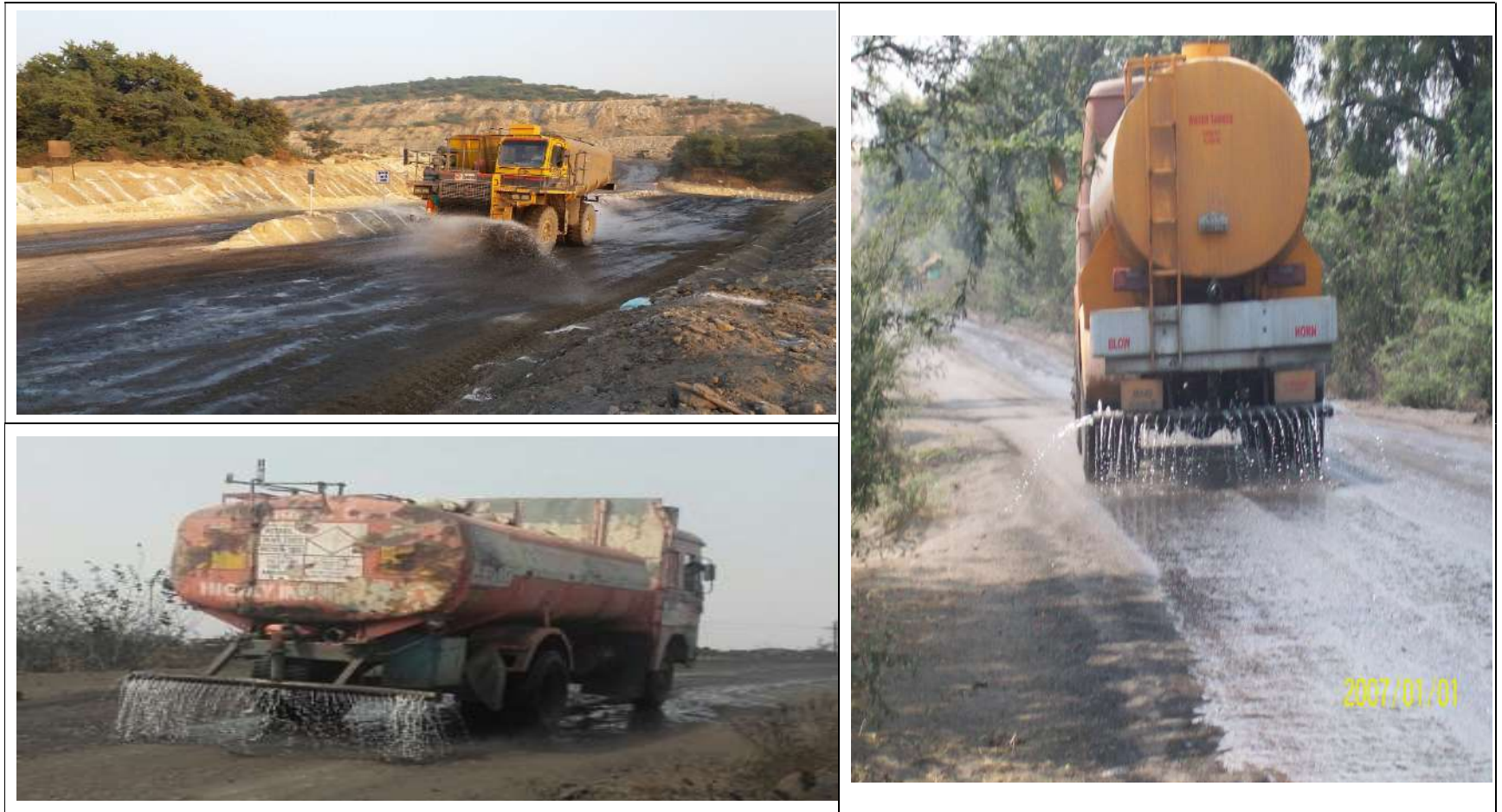
Figure 5 showing water spraying on coal transportation road for dust suppression
