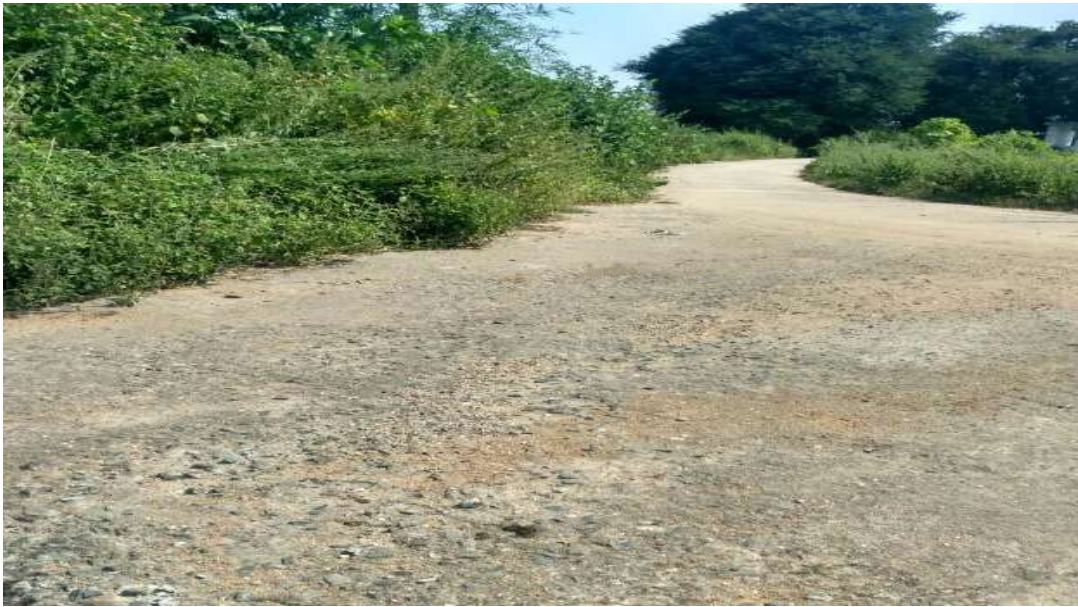
Figure 28 Construction of the cement concrete road from Juni Kamptee to Ghatrohna village
