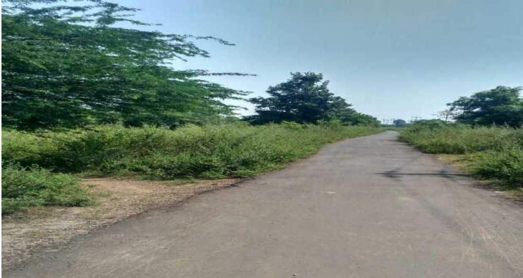
Figure 27 Repairing of the approach road from Yeshamba to Warada village. (Length 400*3m)
