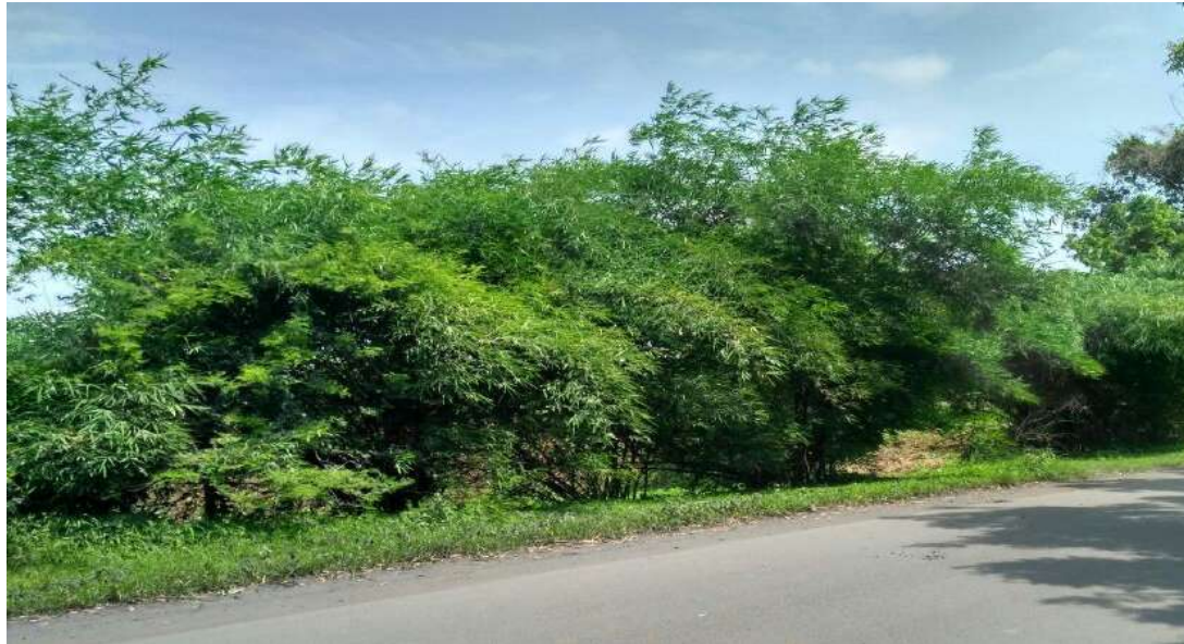
Figure 4 showing Black topped road (length 8.6 Km)
