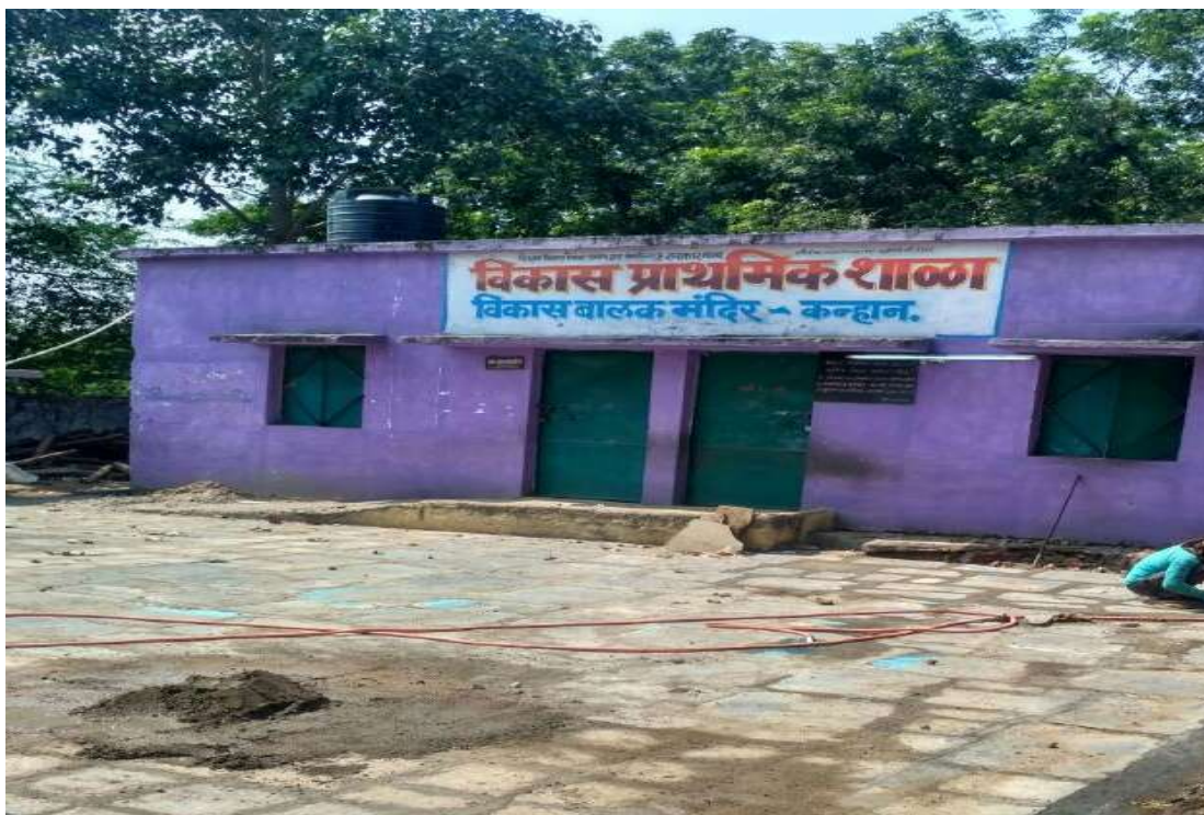
Figure 34 Construction of two rooms at Vikas Prathamik Shala at Kanhan
