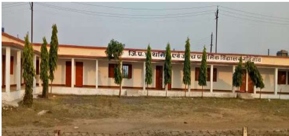
Figure 18 Construction of School Building
