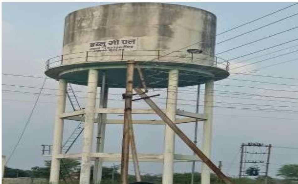
Figure 20 Construction of overhead water storage tank (capacity 2 Lakh litres)
