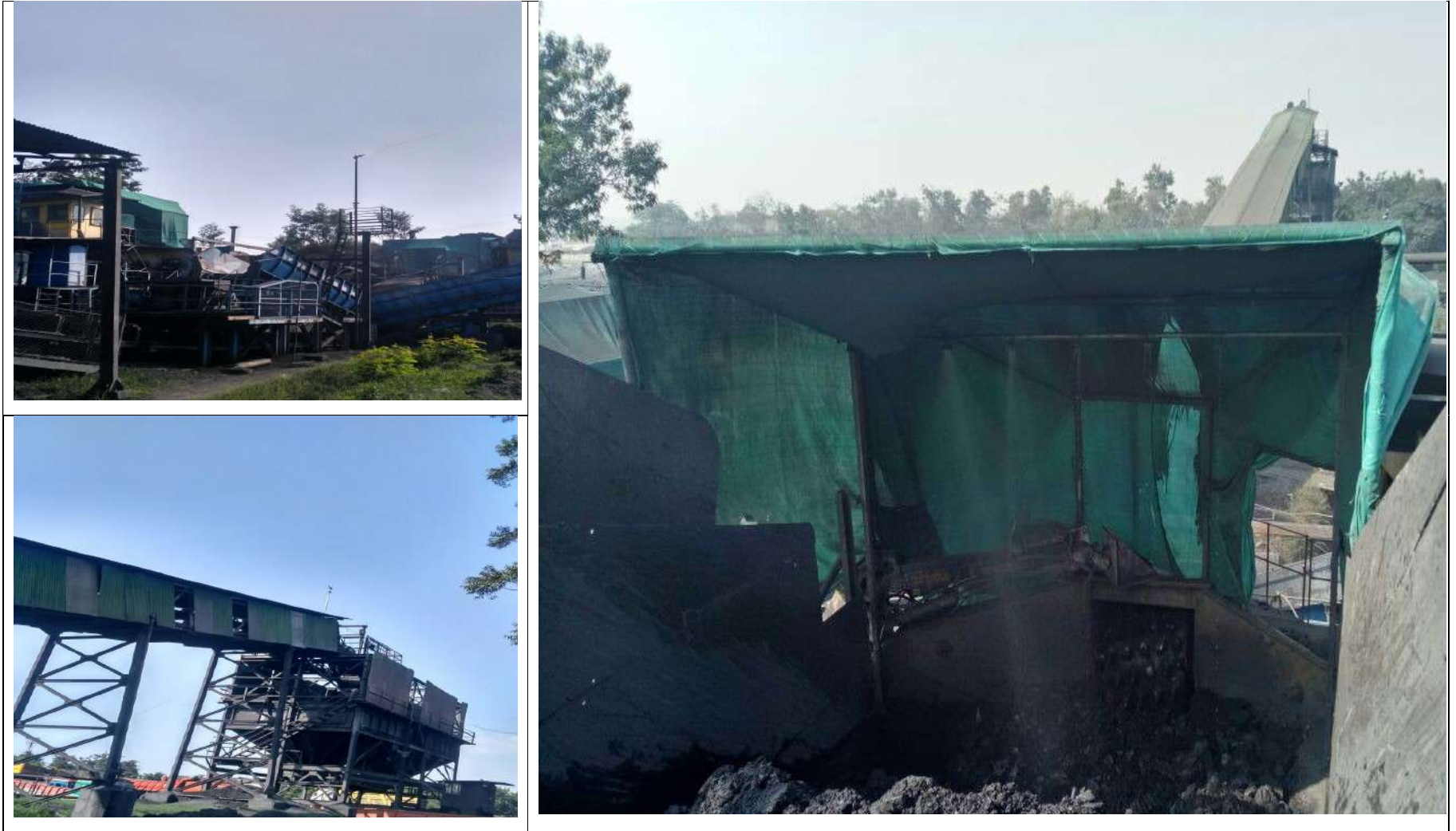
Figure 8 Side Cladding at CHP
