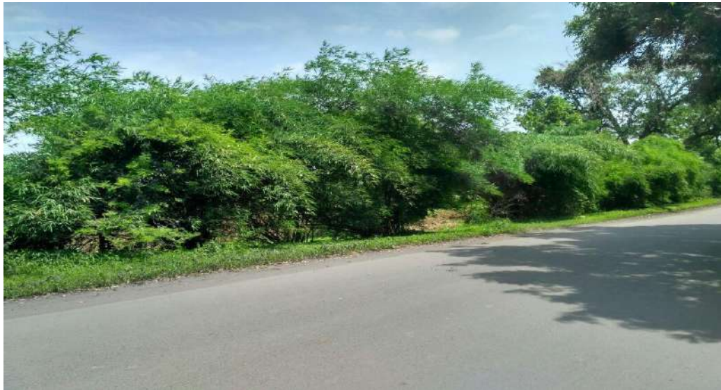
Pic: showing Black topped road (length 8.6 Km)
