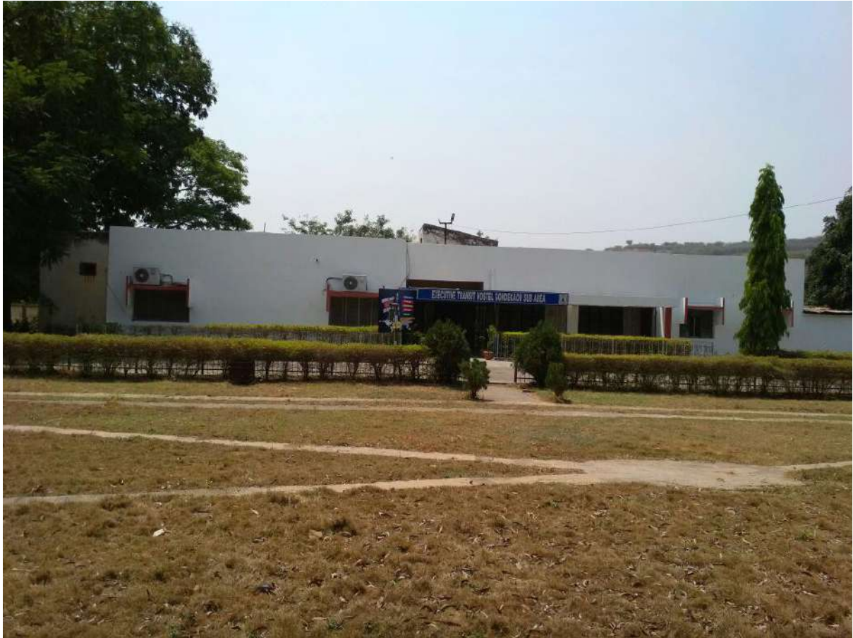
EXECUTIVE TRANSIT HOSTEL AT GONDEGAON
