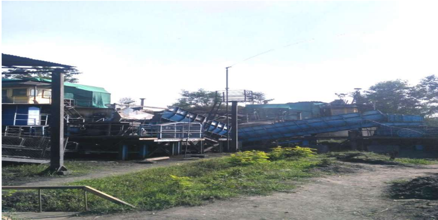
Figure 7 Fixed water sprinkler
