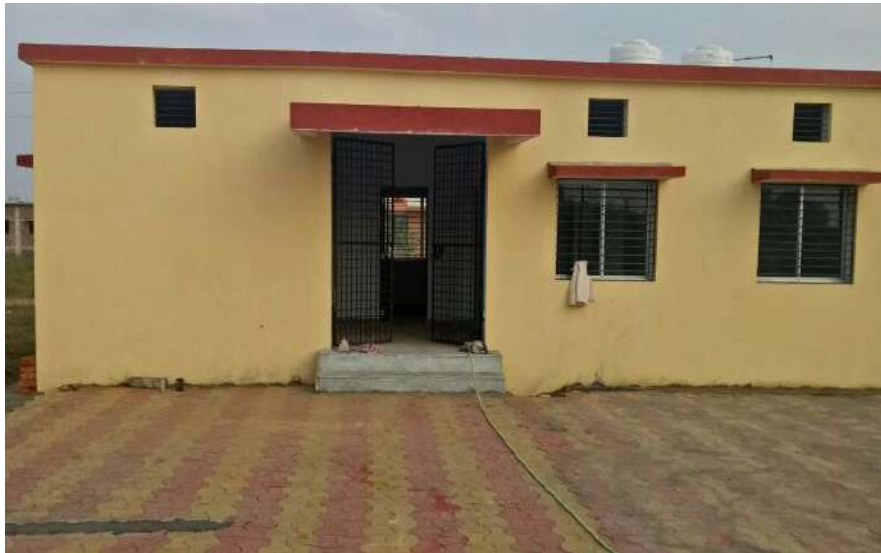
Figure 22 Construction of Public Health Centre
