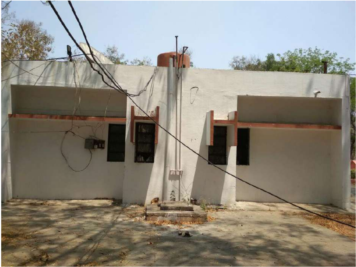
EXECUTIVE TRANSIT HOSTEL AT GONDEGAON
