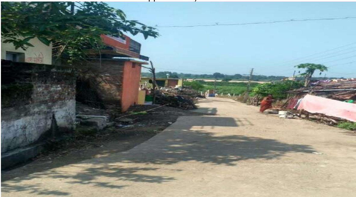
Figure 31 Construction of concrete payment at main road at Yesamba village. (Length 200 m*3.7 m)
