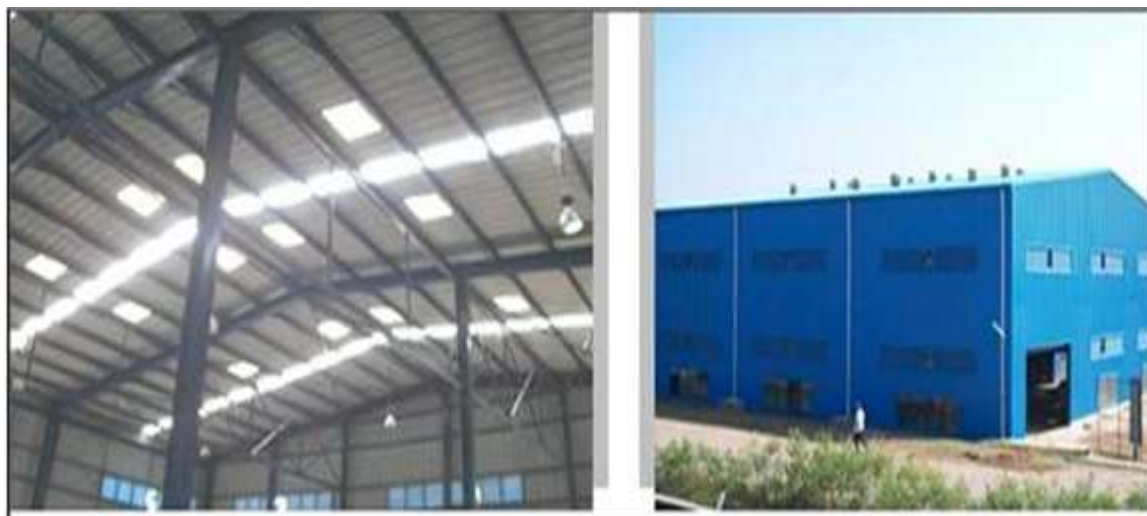
Figure 2-30 : Waste Processing Centre
