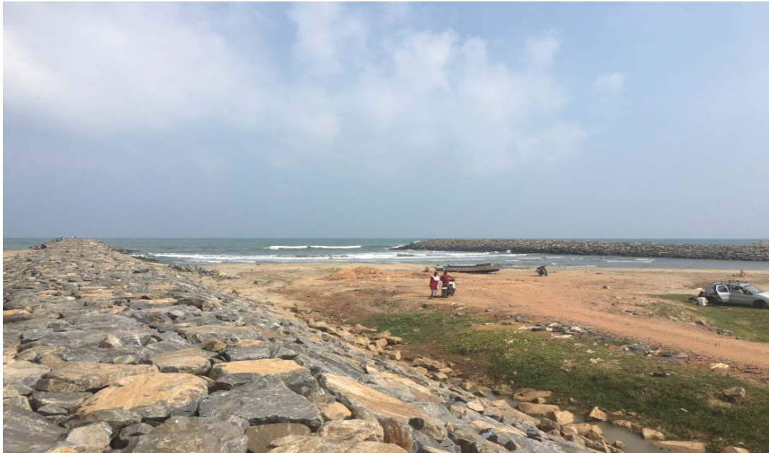
Fig.10.12a View of the pair of training walls at Cauvery confluence point
