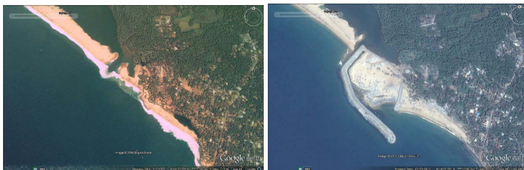
Fig.5.8. Thengapattinam before and after construction of fishing harbour
