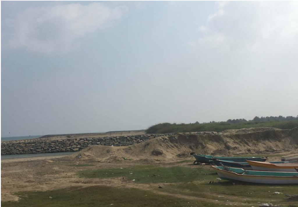
Fig.10.12c View of a groin on the south of Cauvery confluence point
