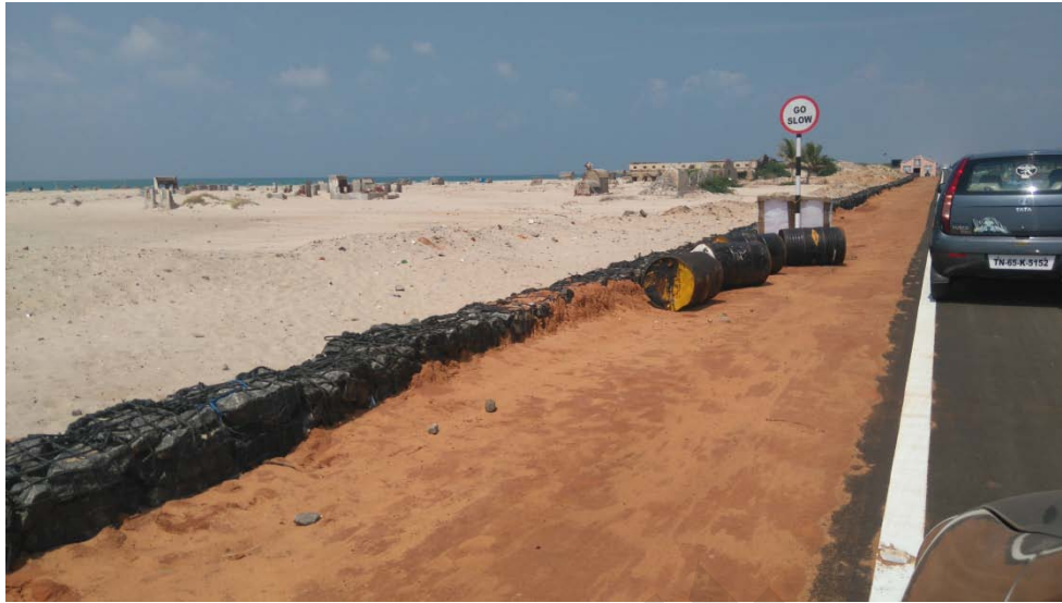
Fig.10.19a. Gabions adopted for protecting the road.
