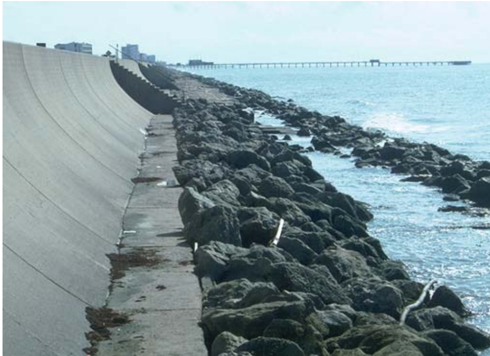
Fig. 1.12 View of a typical concrete seawall
