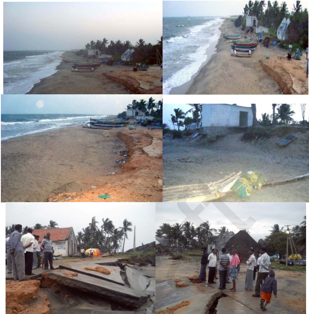
Fig.10.7c Damages along the coast of Devanampattinam
