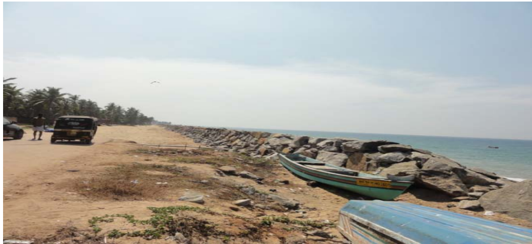
Fig.10.24b Damages to the coastal road
