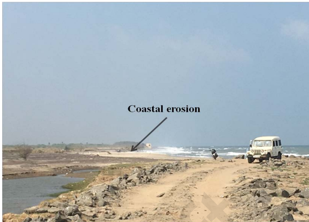
Fig.10.11a View of the eroding shoreline on the north of northern breakwater of Poompuhar fishing harbour. Photo also shows the diverted drainage channel behind the harbour.
