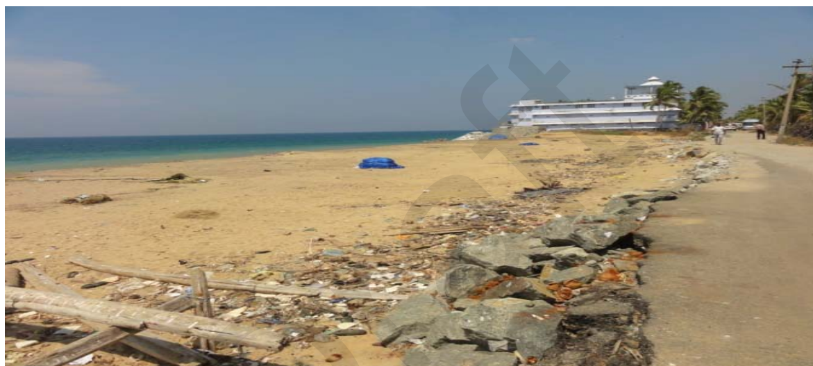
Fig.10.25a Edappadu coastal stretch showing the damages to the coastal road
