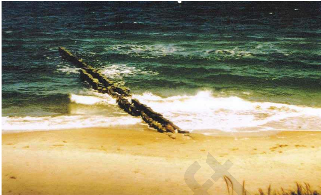
Fig.10.5c Two rows of wooden logs driven into the seabed normal to the shoreline act as groin field.
