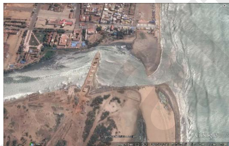
Fig.5.6 Typical view of inlet at Vellar River mouth
