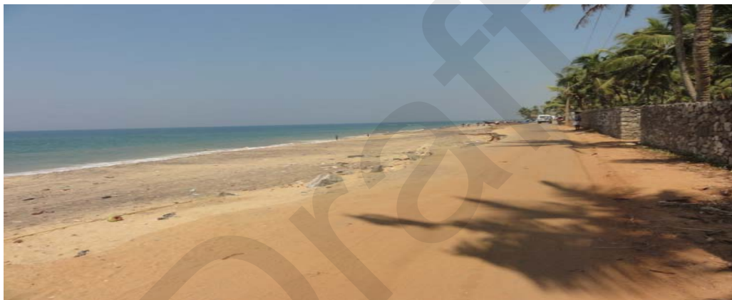
Fig.10.24c View of the partial loss of road width
