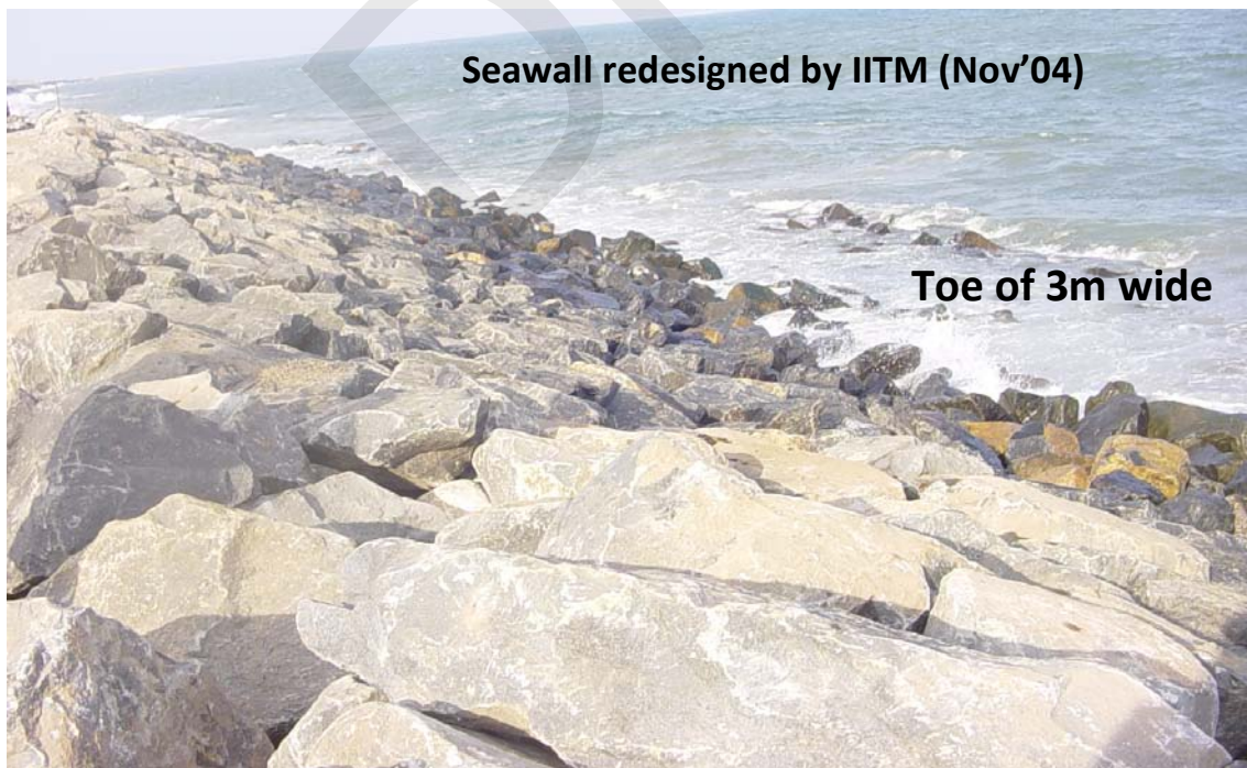
Fig.1.13. Seawall with toe protection north of Ernavur
