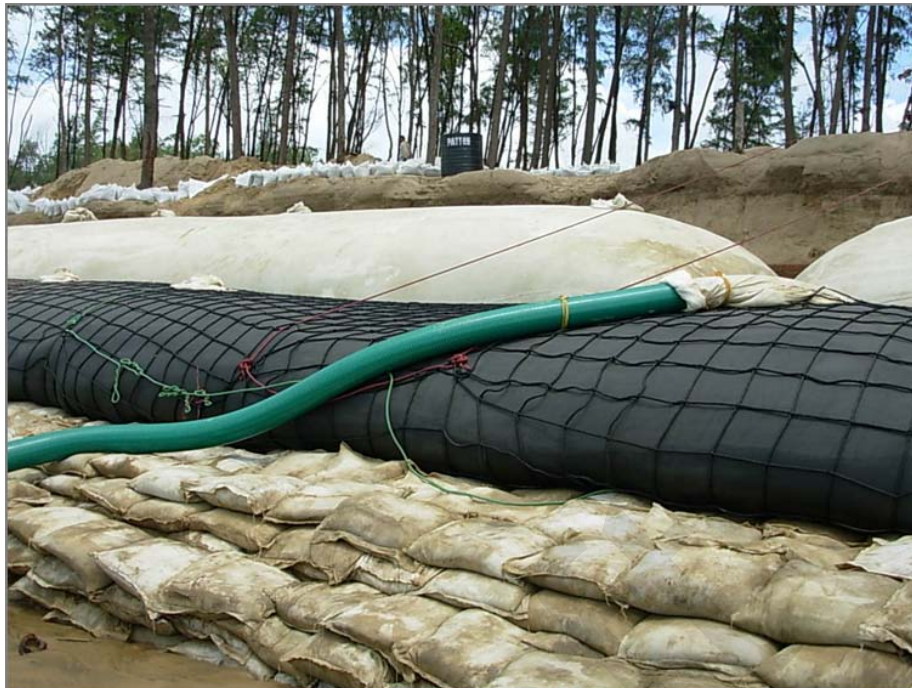
Fig.1.15b Use of Geo-tubes to protect Digha beach, West Bengal (IITM)
