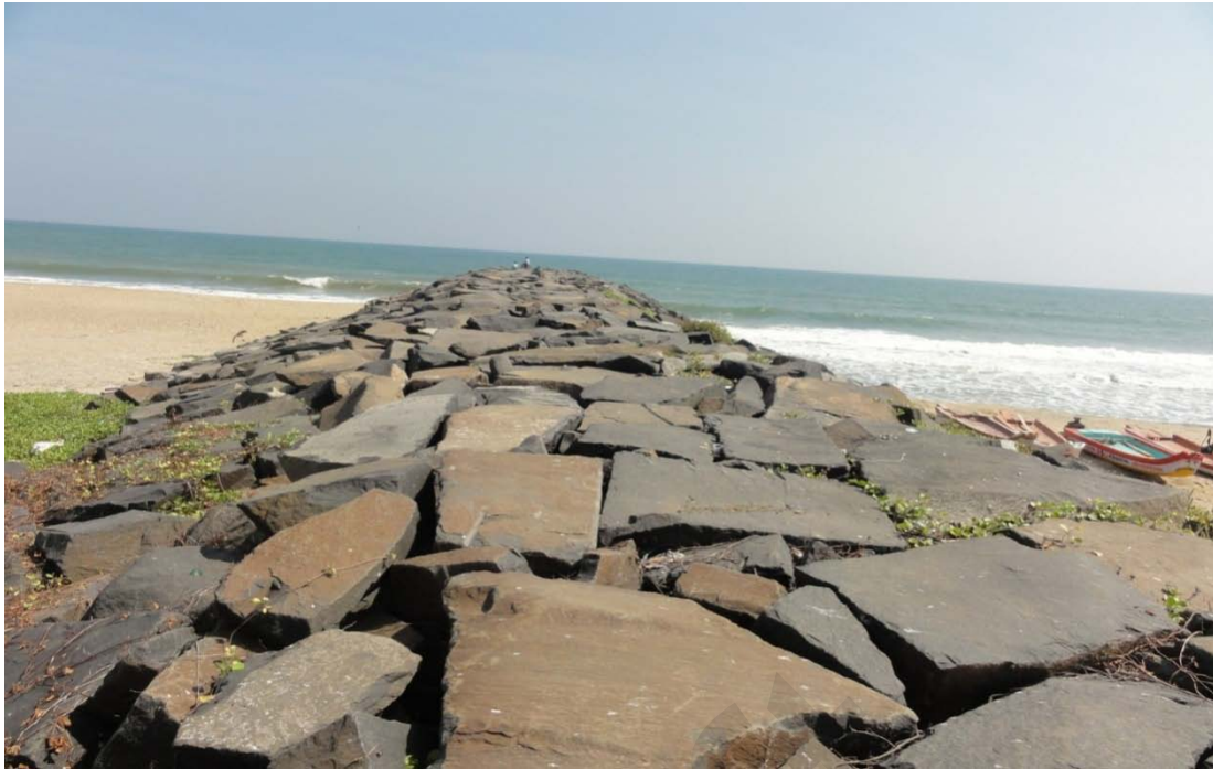
Fig.10.6 Trunk of the groin
