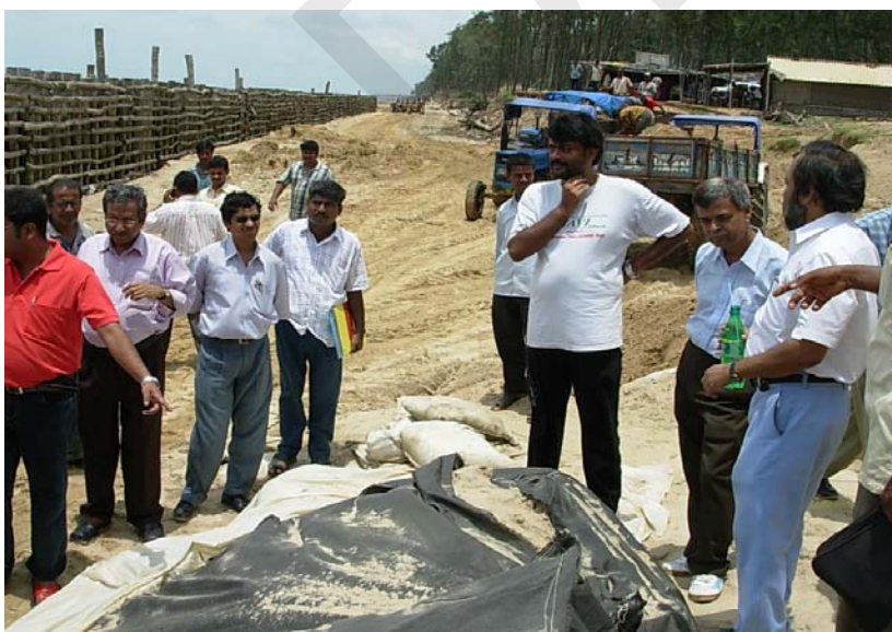
Fig.1.35bvandalism-punch ring of geo-tubes
