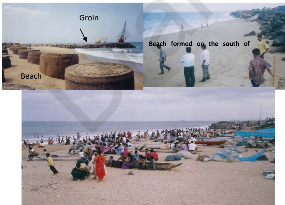
Fig.1.23. Effect of Groin field in winning the beach (Royapuram, Chennai)
