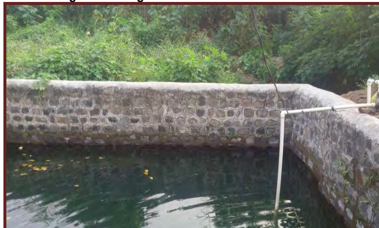
Figure 3.7: Dug well on nalla bank in Thakurwadi
