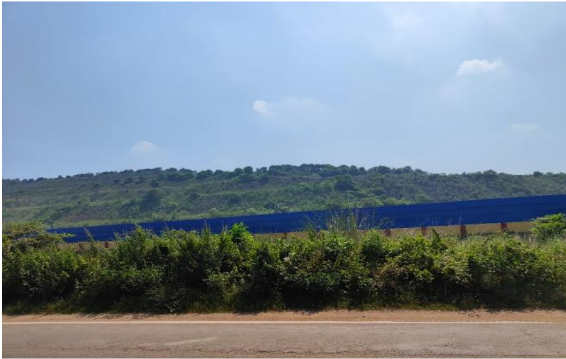
Vertical Wind Barrier along Railway Siding at Sonapur Bazari Area
