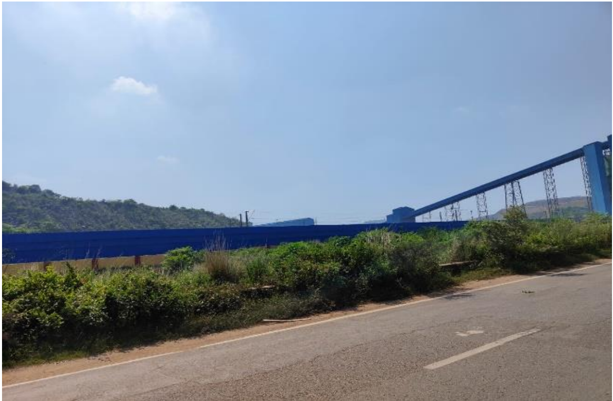
Vertical Wind Barrier along Railway Siding at Sonepur Bazari Area
