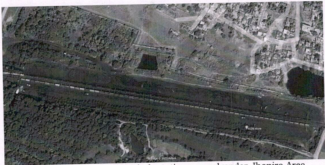
POCP 1 Railway Siding and plantation around under Jhanjra Area
