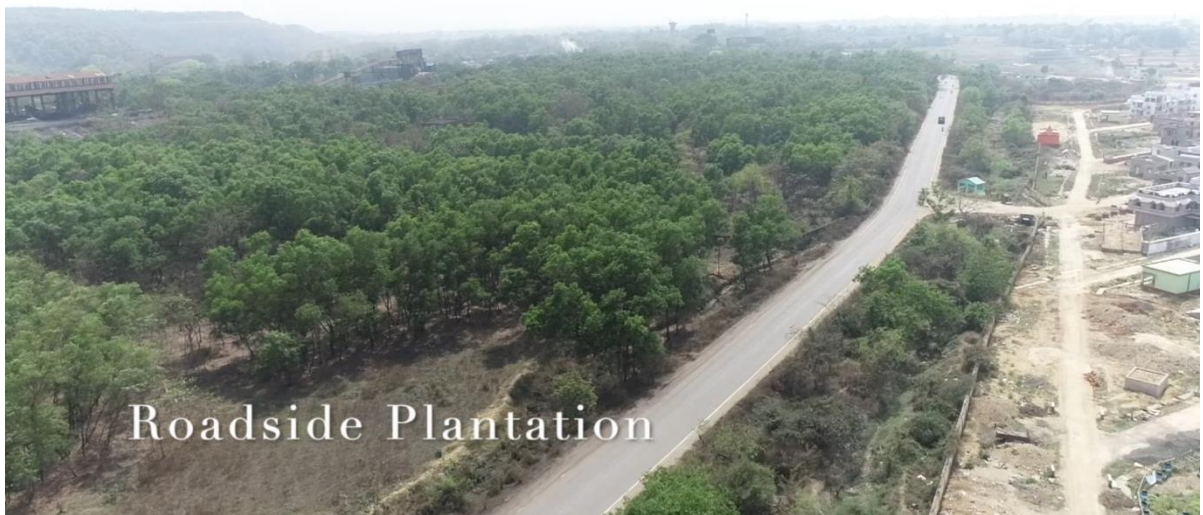
9 Ha Road Side Plantation around NH 60 under Sonapur Bazari Area
