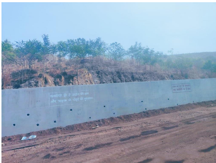
Toe Wall Constructed at OB Dump
