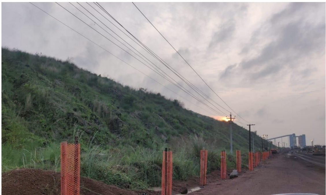
Road Side Plantation along with tree guard at Sonapur Bazari Area
