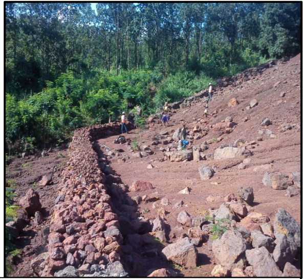
Proper retaining wall provision at the bottom peripheral of the dump
