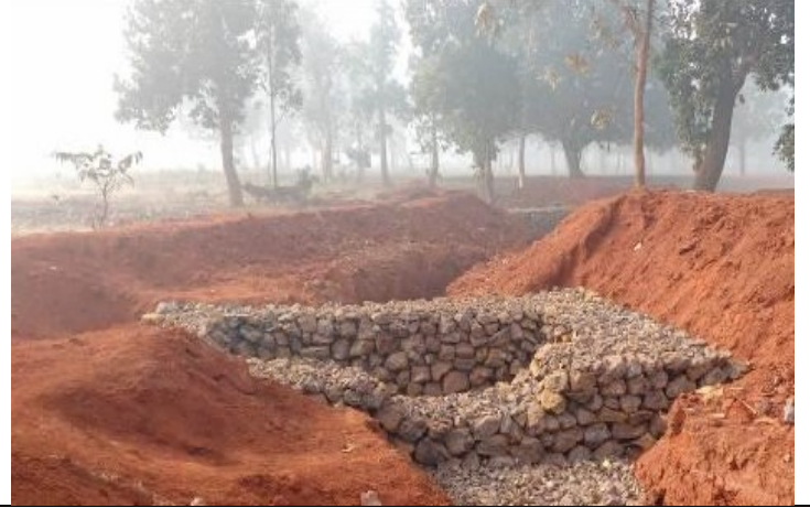
B. Check weir at Gangeigoda
