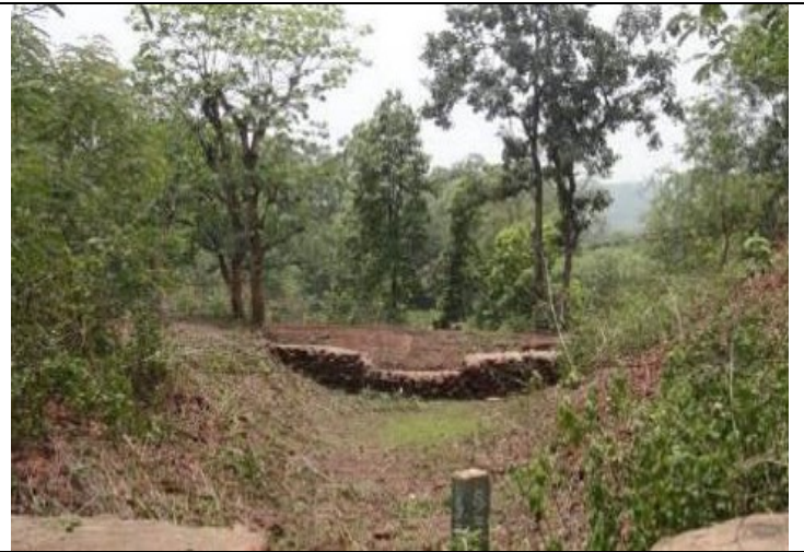
Check weir at Udalbadi
