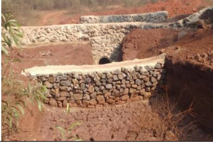
Check weir at Barpada
