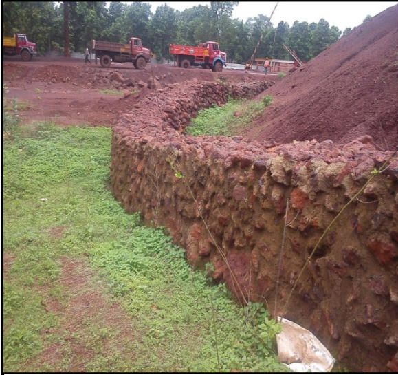
Proper retaining wall provision at the bottom peripheral of the dump
