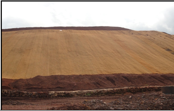
RETAINING WALL PROVIDED AT THE TOE OF THE DUMPS
