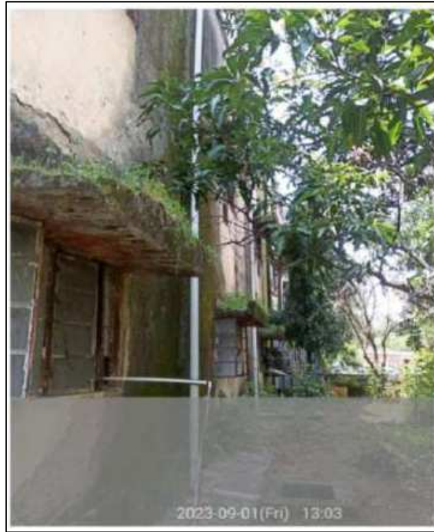
Figure 15: Existing rain water harvesting at Regional Workshop, Pathakhera Area, WCL
