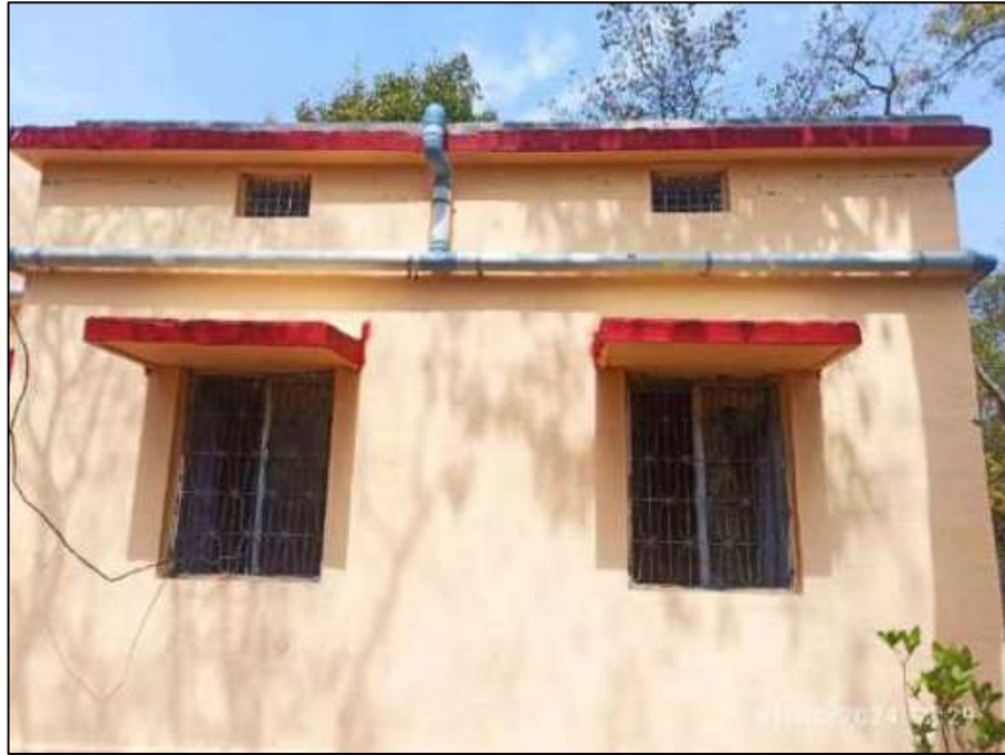
Figure 17: Existing rain water harvesting at Office Building, Tawa UG Mine, Pathakhera Area, WCL.
