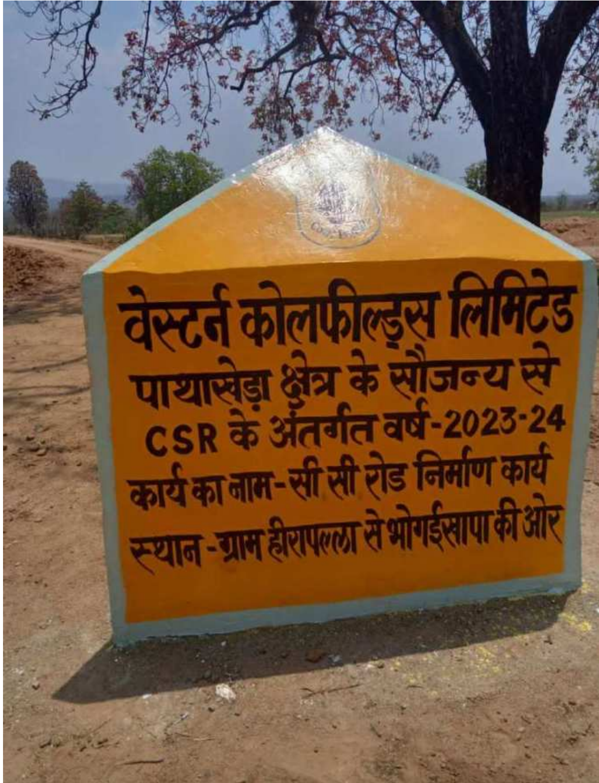
Photos of RCC Road built in Hirapalla – Bhogaikhapa village under CSR Activities during FY 2023-24
