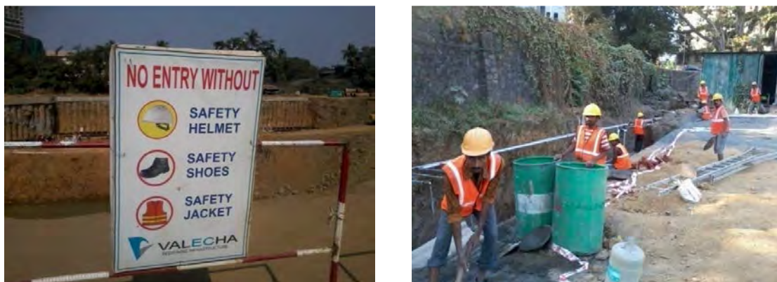
Plate3.3: Safety Implemented at Project site
