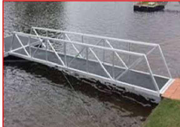
Figure 2.6: Typical Access Gangway (Aluminium)
