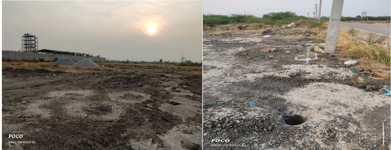
FIGURE-1.4: PHOTOS OF THE PROJECT SITE
