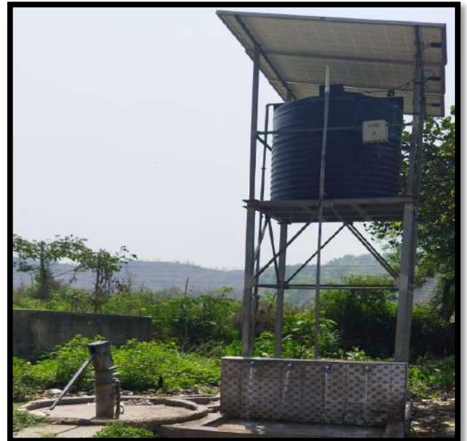
Deep Borewell at Kathara OCP
