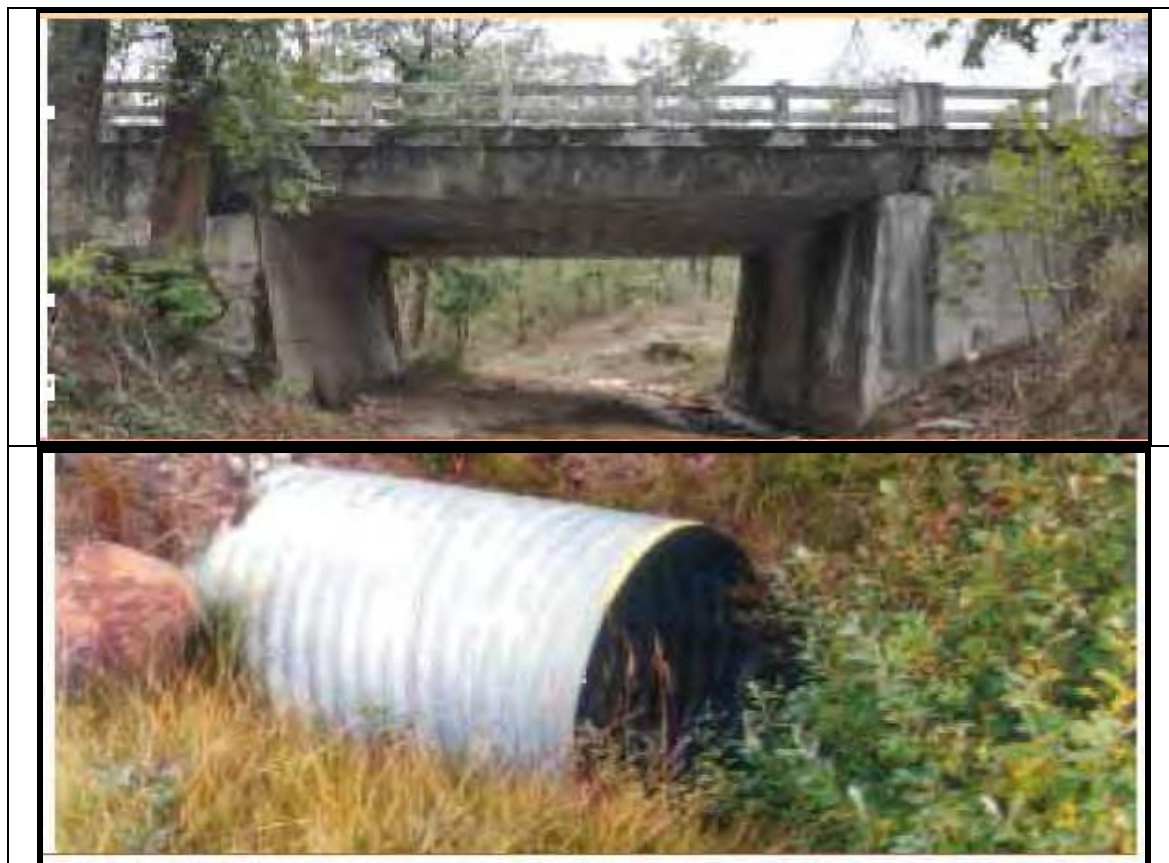
Figure 5.4: Suggestive engineering devices for wildlife management (WII 2016) Top-underpass, Middle-Box culvert; Lower-Pipe culvert
