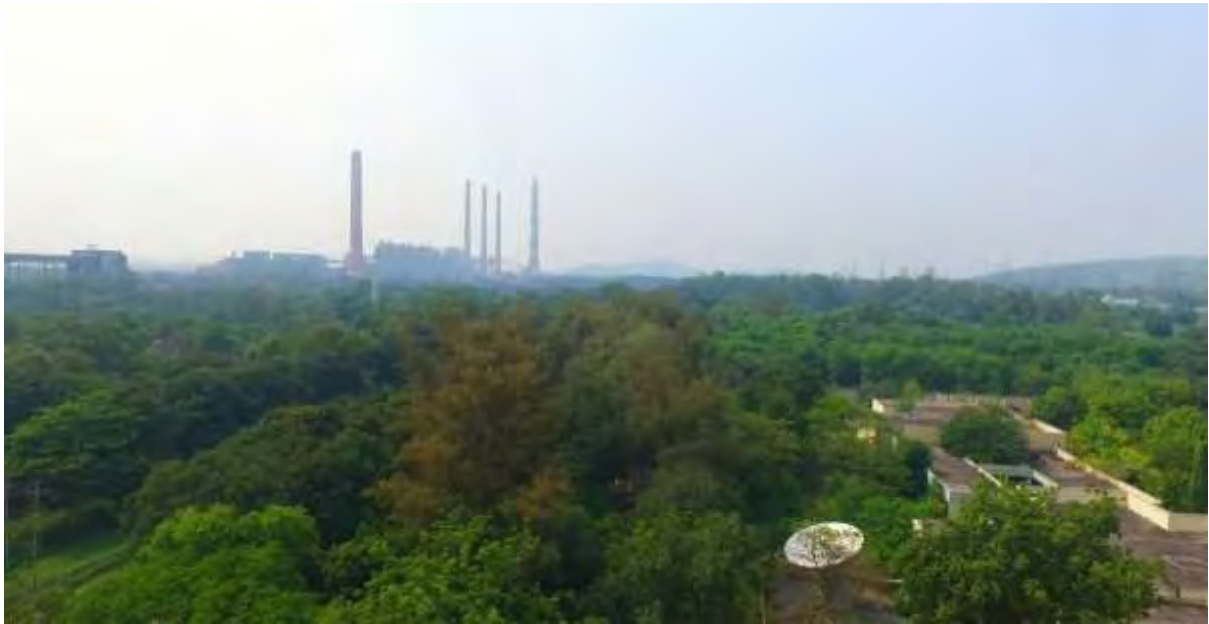
OVERALL VIEW OF PLANTATION WITHIN PLANT AREA
