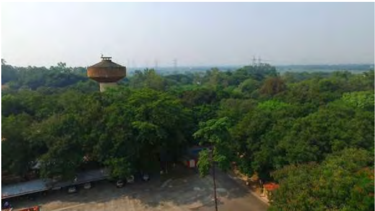
NEAR EMPLOYEE DEVELOPMENT CENTRE (EDC)
