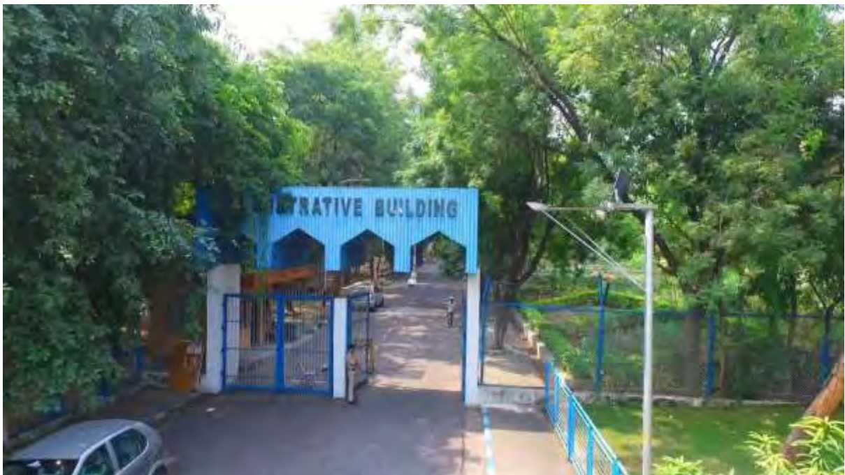
NEAR ADMINISTRATIVE BUILDING ENTRANCE
