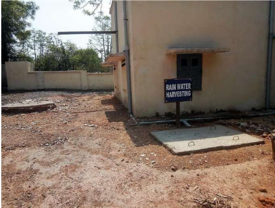
Fig: Rain Water Harvesting Structure at PO Office
